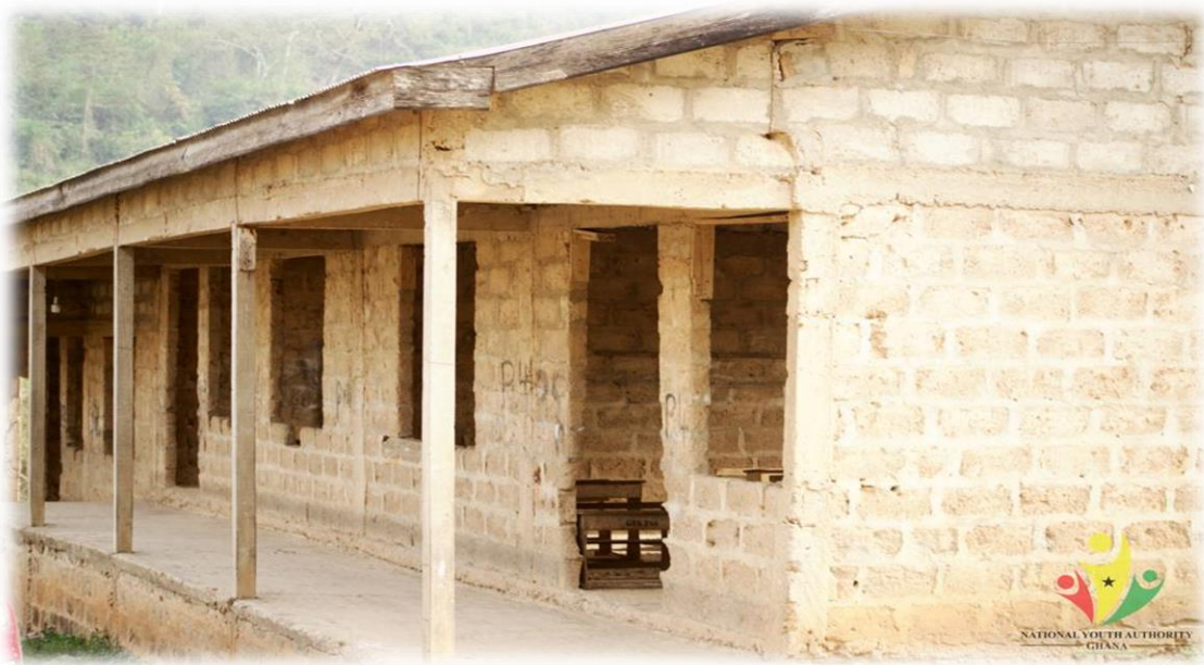
Before Renovation of classroom block
