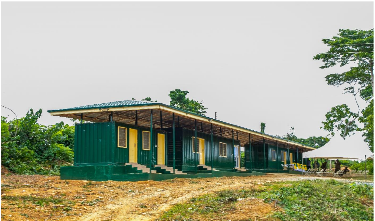
Construction works at the Tactical Training Grounds, Kyebi, Eastern Region (100% completed)
