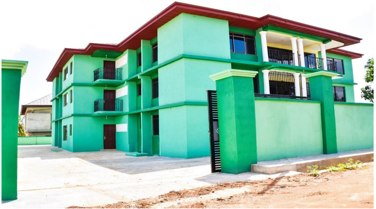
Refurbishment of 9 units, 2bedroom residential accommodation at Buokrom, Ashanti Region (Entrance) (100% completed)
