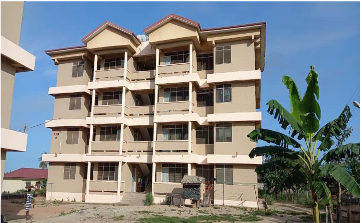
4-storey 8 unit block of three/3 bedroom flats completed
