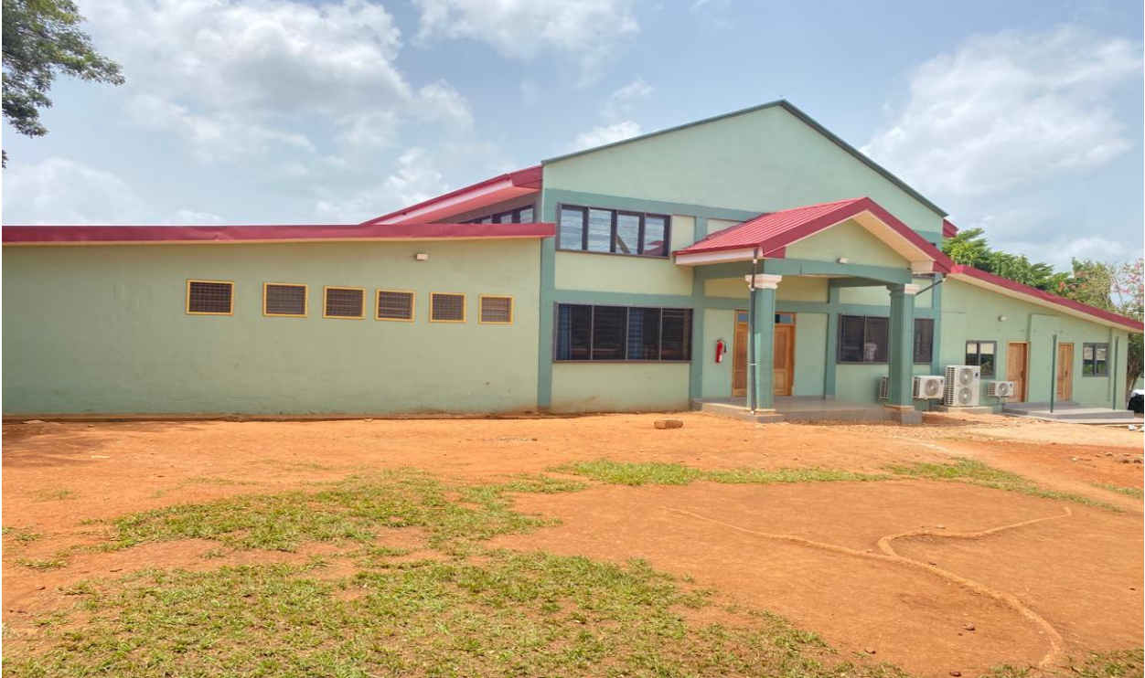
Refurbishment of Lecture Hall and Administration Block
