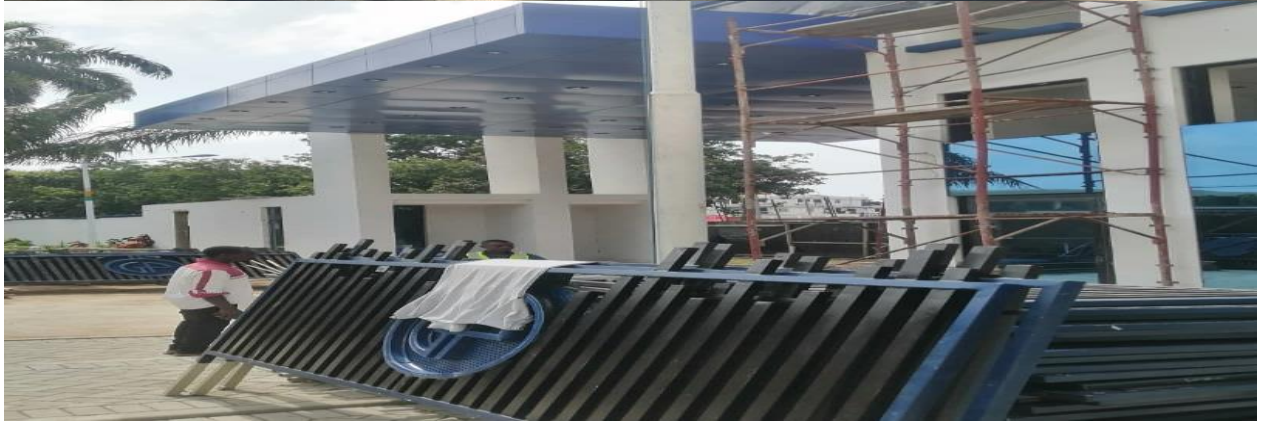
The new Ghana Police Service Headquarters main entrance
