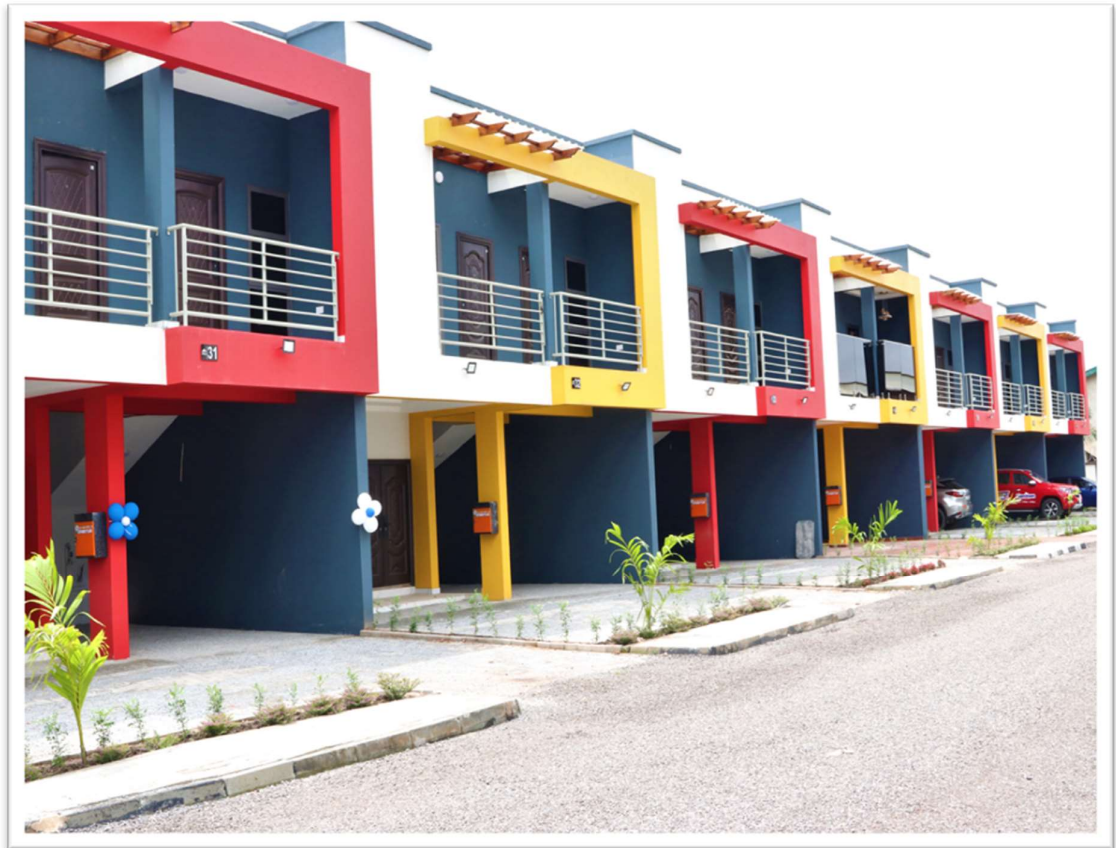
Figure 4: Legacy Court Housing Project
