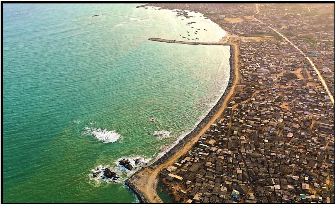
Figure 6: Aboadze Coastal Protection Project (Phase II)
