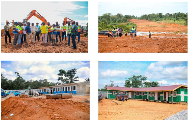
Accra – Kumasi Bypass Project – Site Clearing
