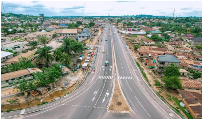
Assin Praso-Assin Fosu road project
