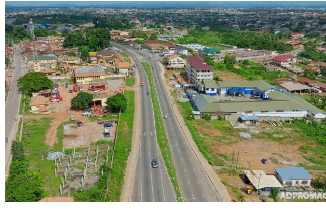
Kumasi Lake Road and Drainage Extension Project
