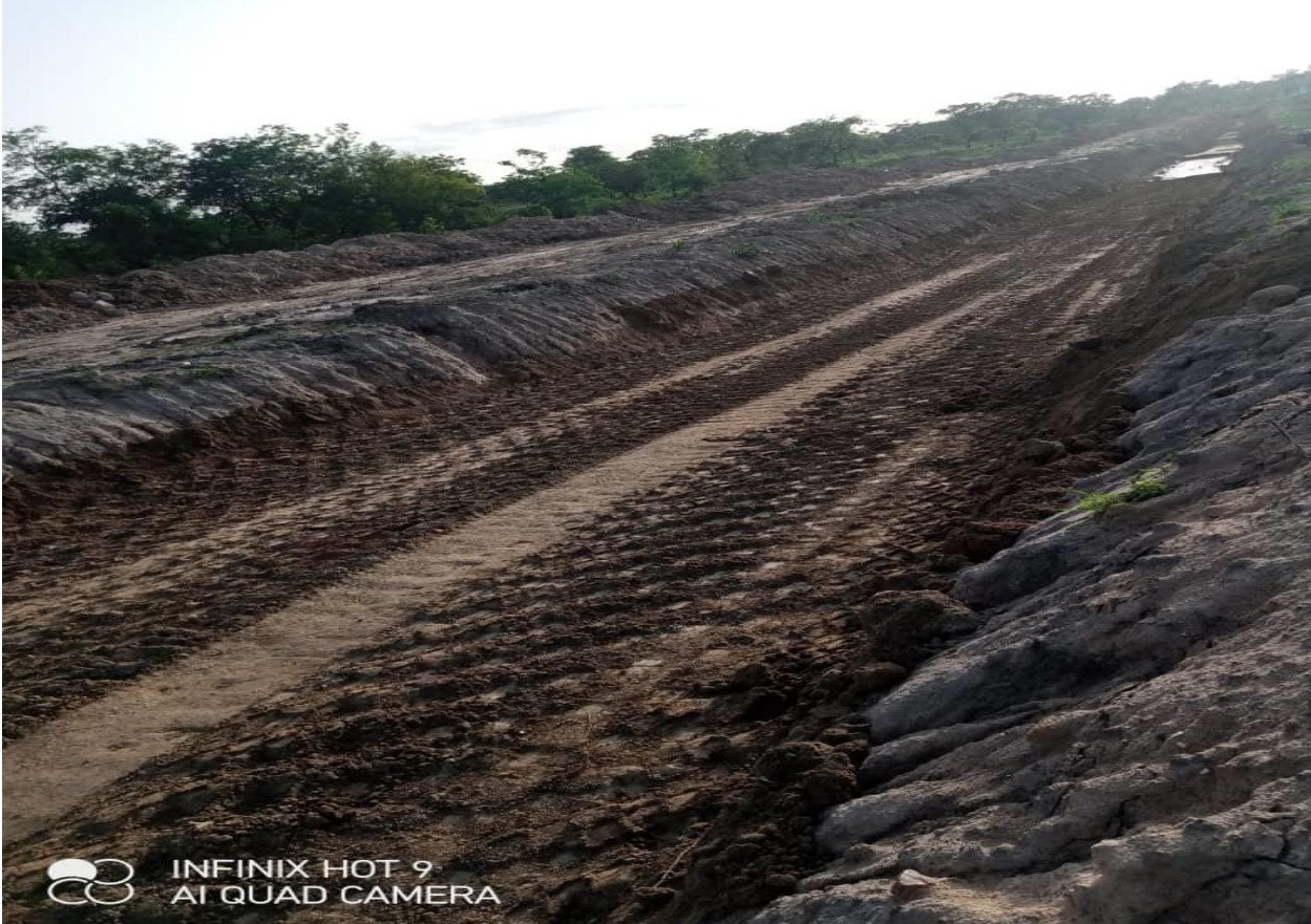
Key trench excavation
