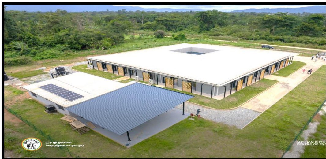
Figure 10: Newly Constructed TVET Centre of Excellence At Anyinam
