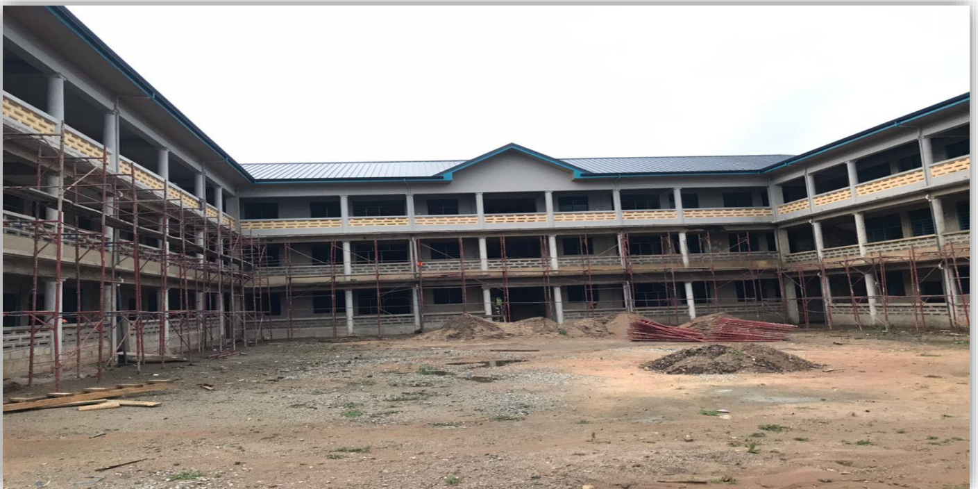
3 Storey 12x Chamber & Hall Bedroom Flats at Air Force Base Accra
