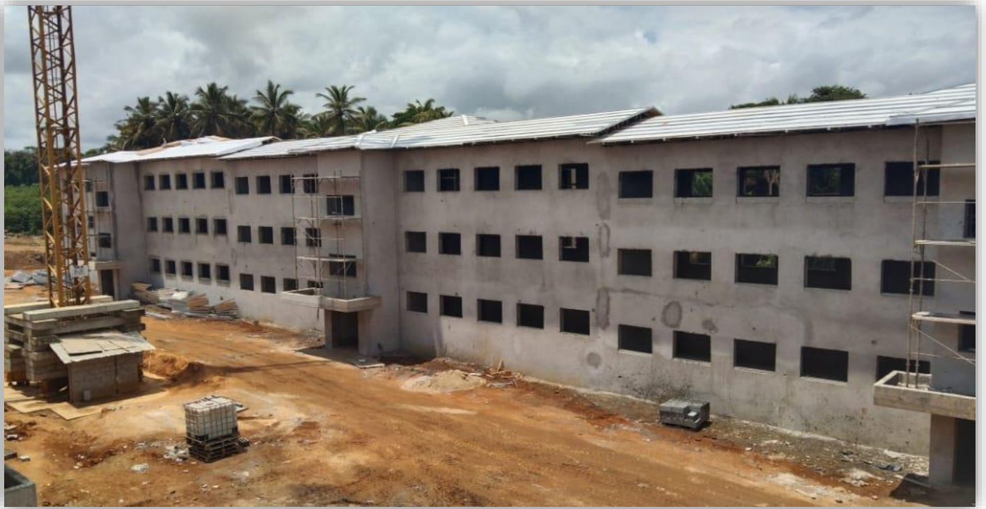
Construction of accommodation facilities at Forward Operating Base (FOB) at Ezinlibo
