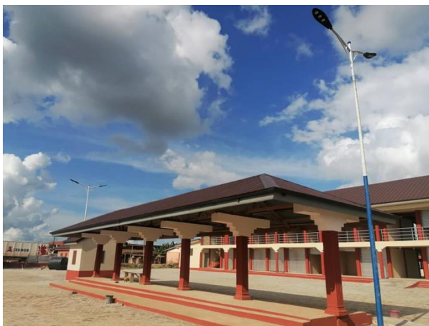
Construction of 7No. 20-Unit Stalls, at Berekum East MA
