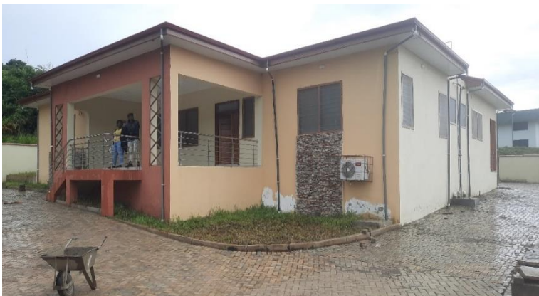
ERECTION AND COMPLETION OF 2NO SENIOR STAFF BUNGALOWS FOR GHANA HEALTH SERVICE AT WORAWORA
