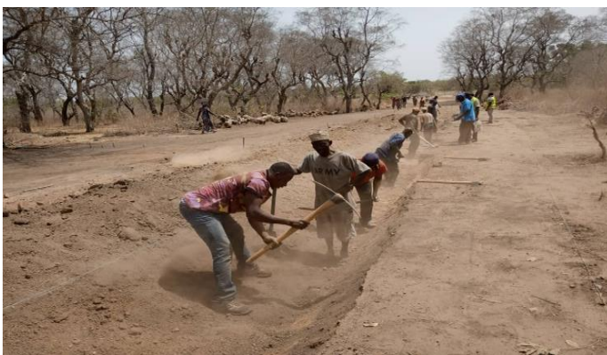
Lipw Feeder Road Formation At Boya-Adonsi-Adagbira In Bawku West District
