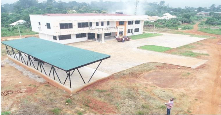
CONSTRUCTION OF 2-STOREY ADMIN BLOCK FOR DEPT. OF AGRIC AT GOASO
