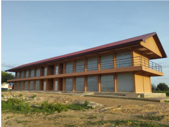
Construction of 1 No. 2-Storey 40-Units Lockable Stores and Fire Post at Tindonsobligo –Kalebeo, Bolgatanga at Bolga MA
