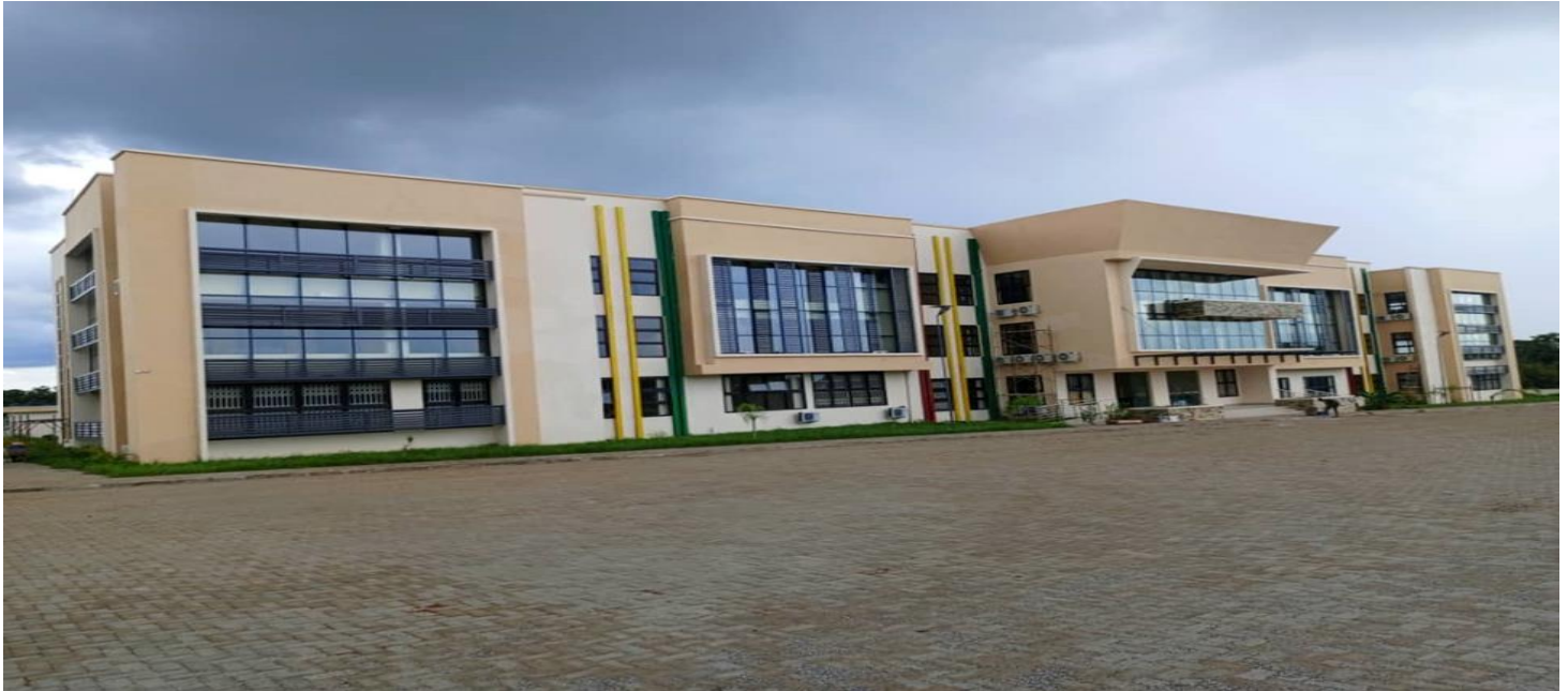
COMPLETION OF 1 NO. 3-STOREY ADMINISTRATION BLOCK FOR SAVANNAH REGIONAL CO-ORDINATING COUNCIL (RCC) AT DAMONGO
