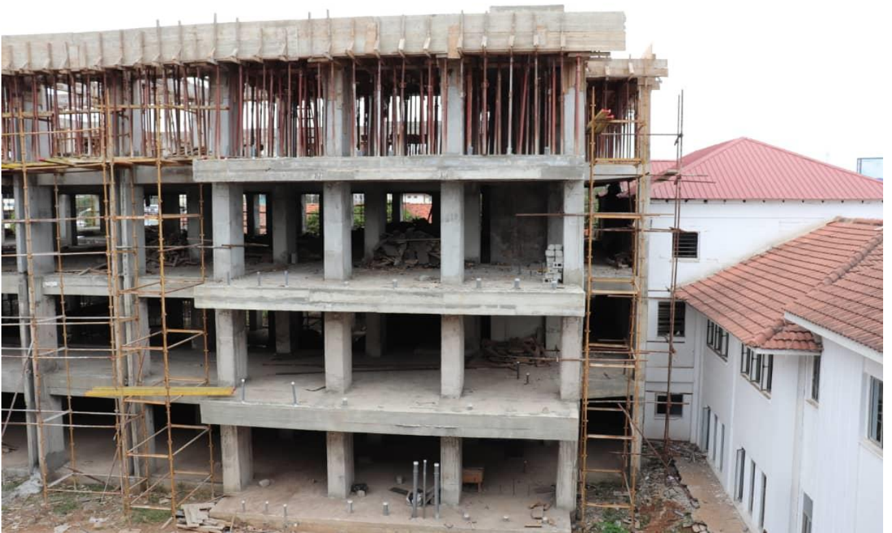
Reconstruction of burnt section of the Old Parliament House – WIP
