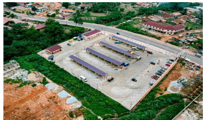
Kumasi Lake Road and Drainage Extension Project – Dompouse Lorry Terminal
