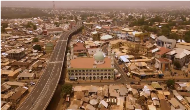
Tamal Interchange (Sinohydro Project)
