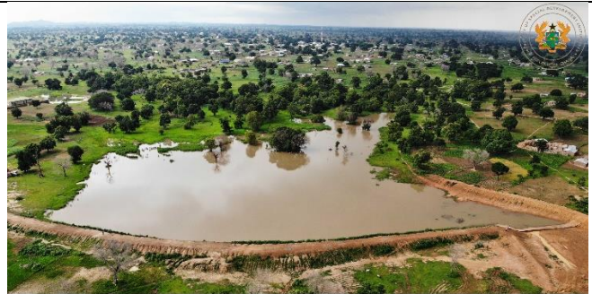
SMALL EARTH DAM, MANYORO, NAVRONGO, UPPER EAST
