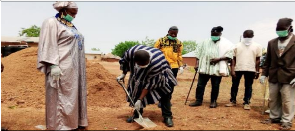
Sod-cutting Ceremony for Construction of Maternity block project for in Tolon Constituency
