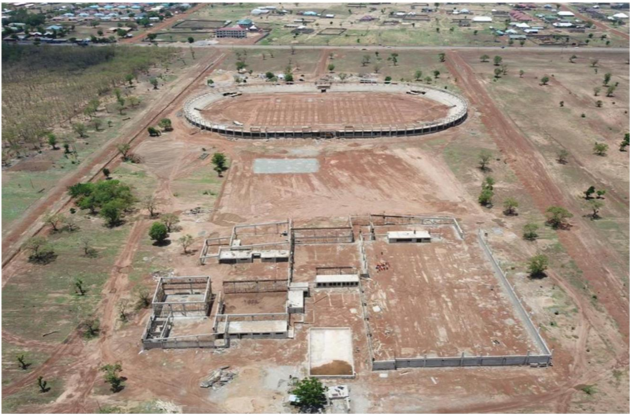
Construction of GAF Sports Centre at Tamale
