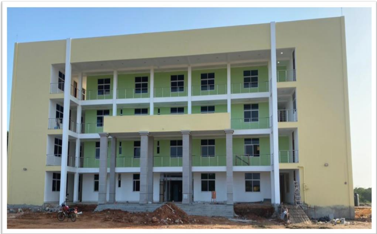
An ongoing section of the building
