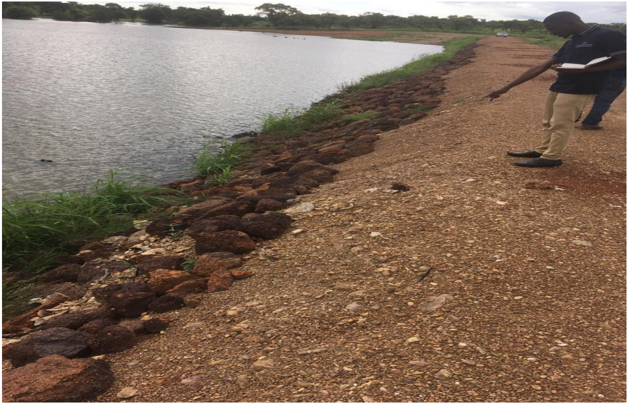
Completed Small Earth Dam at Dagri in the Upper West Region
