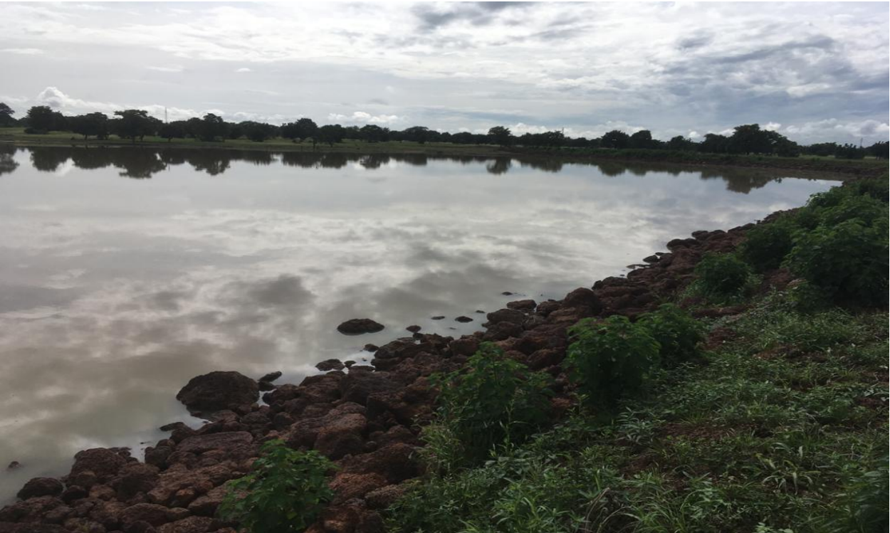
Completed Small Earth Dam at Tokun in the Upper West Region
