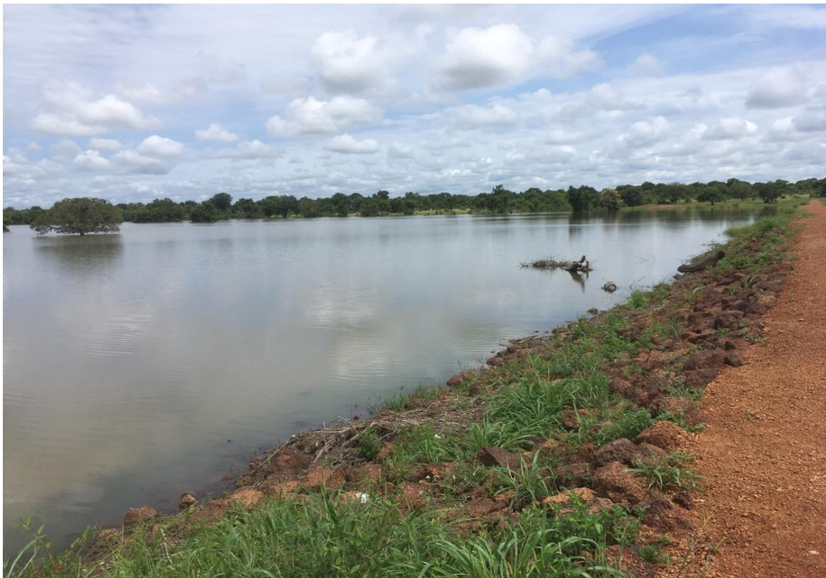
Completed Small Earth Dam at Sentu in the Upper West Region
