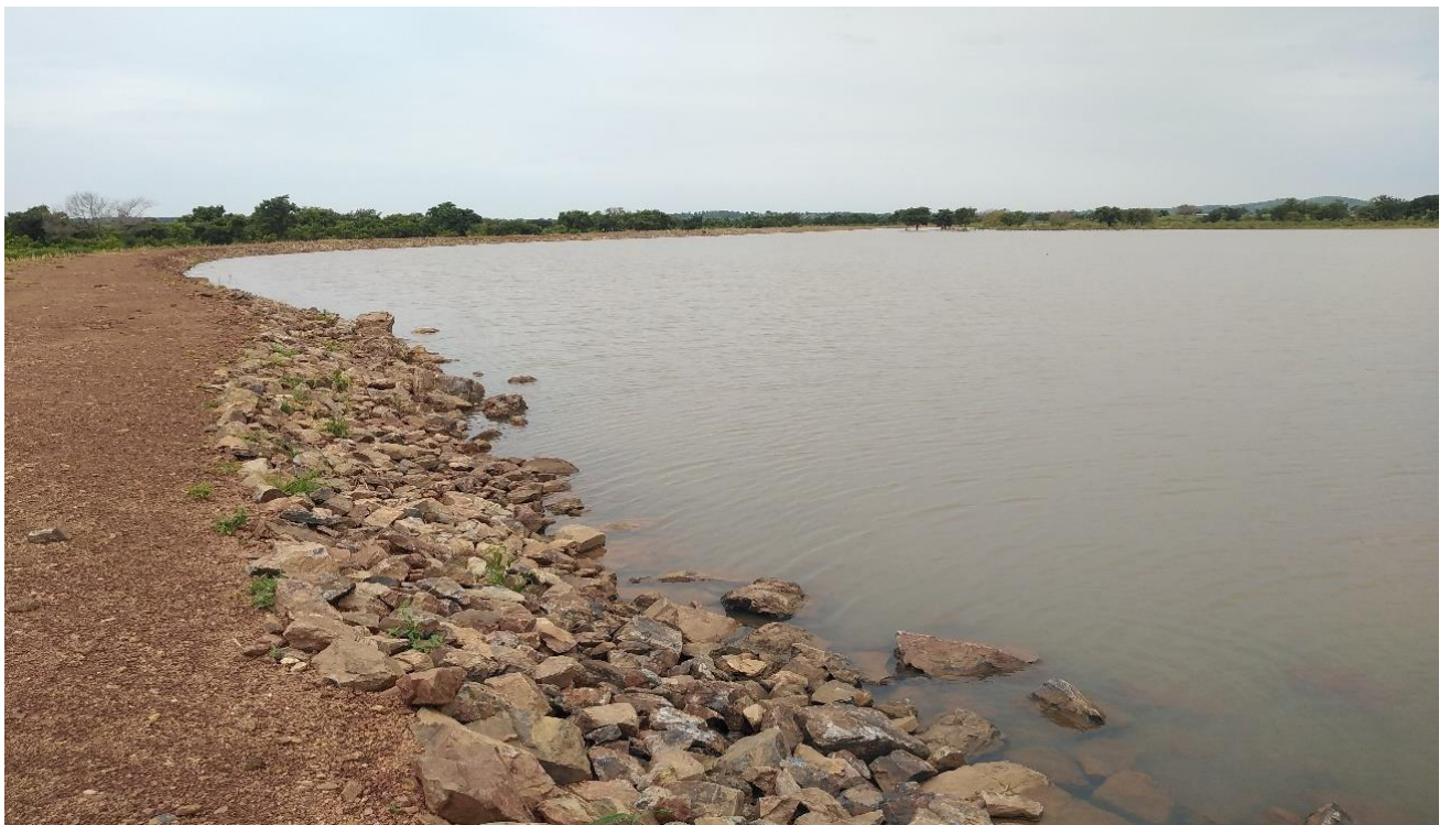
Completed Small Earth Dam at Namolgu in the Upper East Region
