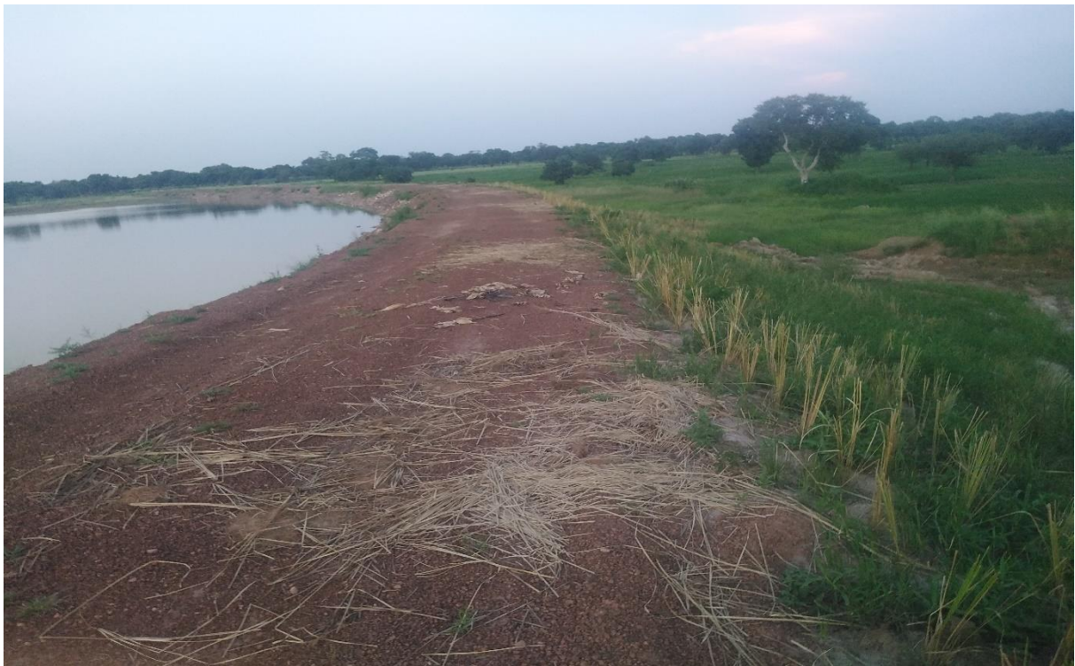
Completed Small Earth Dam at Vunania in the Upper East Region
