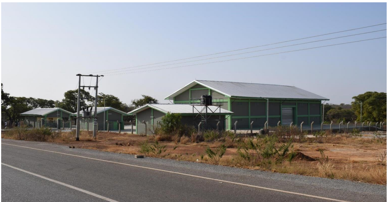
Completed warehouse with ancillary structures at Bussie in Upper West Region
