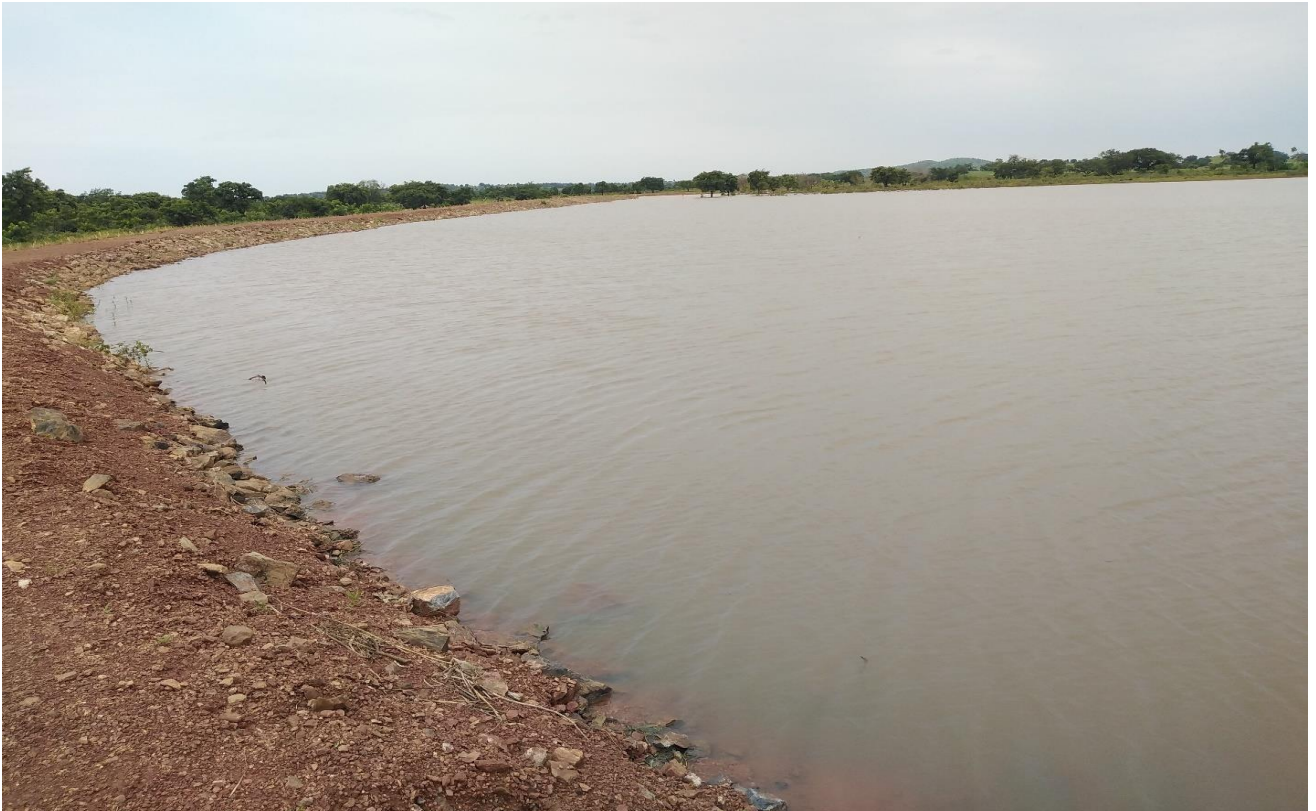
Completed Small Earth Dam at Namolgu in the Upper East Region
