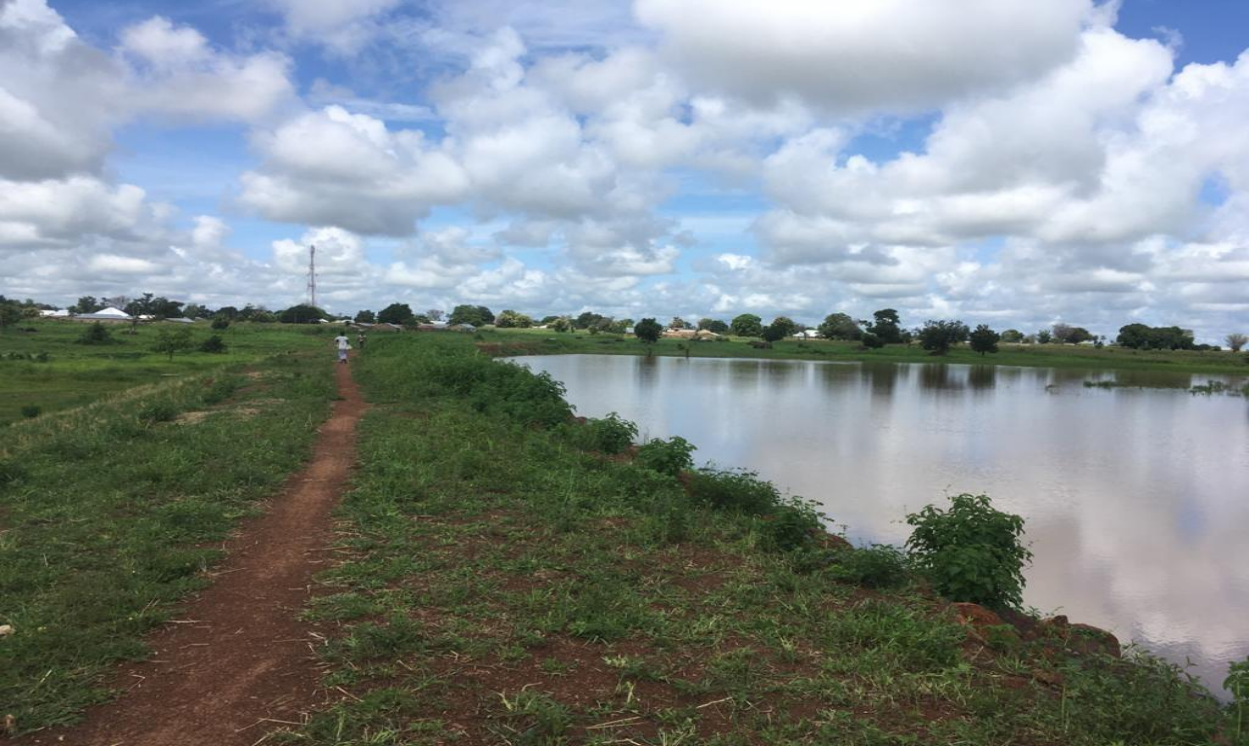
Completed Small Earth Dam at Tuopare in the Upper West Region
