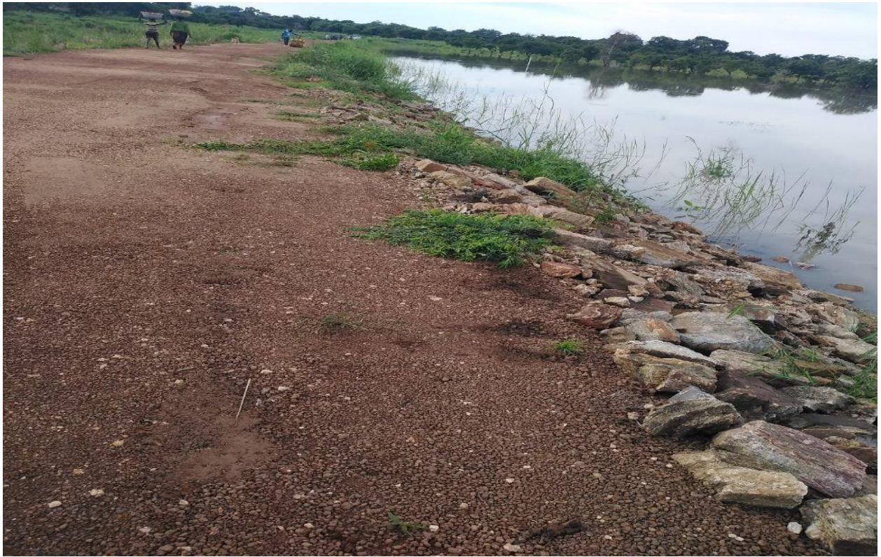
Completed Small Earth Dam at Duong in the Upper West Region
