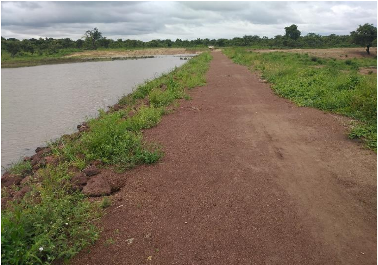
Completed Small Earth Dam at Kataa in the Upper West Region
