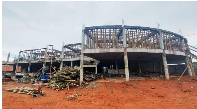
GARO Phase II Under Construction
