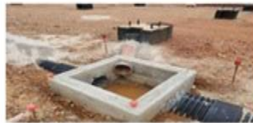
Figure 3: Inspection Chamber, Storm Water
