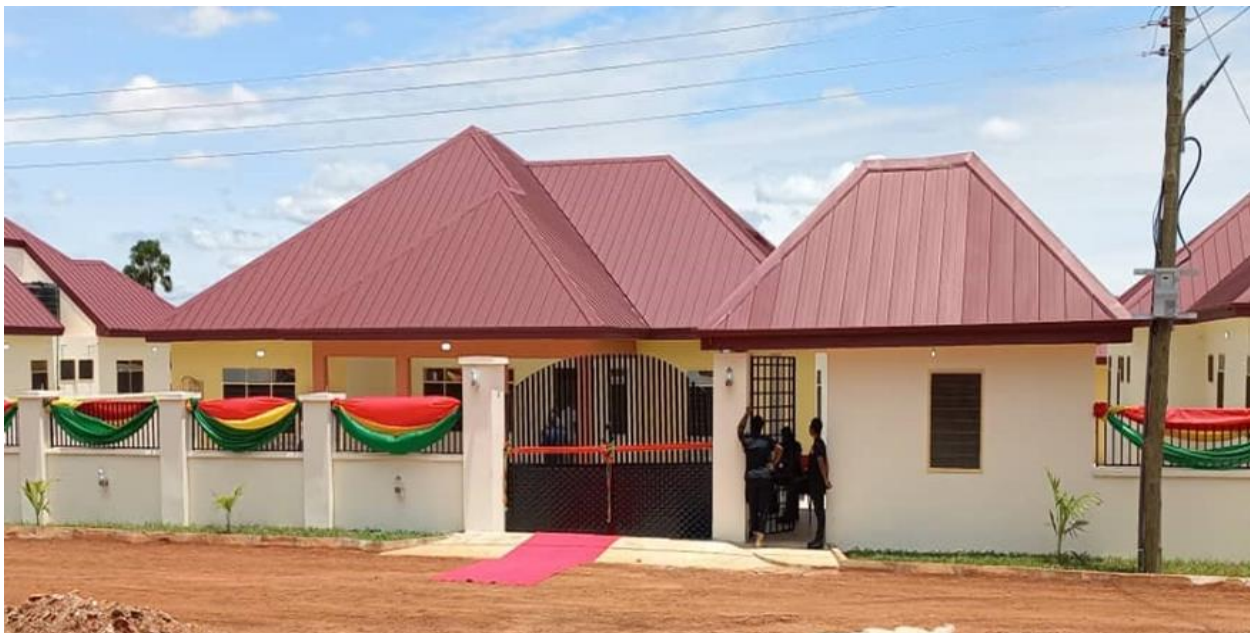
COMPLETED 3NO. SENIOR STAFF BUNGALOWS FOR STAFF OF THE BONO EAST REGIONAL COORDINATING COUNCIL (BERCC) AT TECHIMAN, BONO EAST REGION
