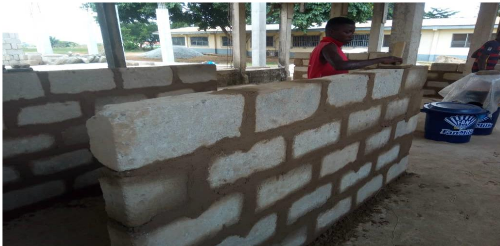
Masonry practical demonstration at CDVTI- WA
