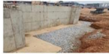
Figure 2: Sub-structural Works, Retaining Wall
