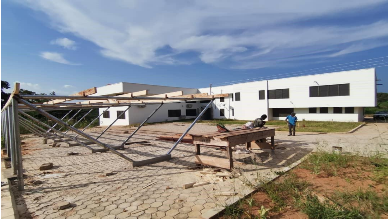
COMPLETED 1NO. 2-STOREY ADMINISTRATION BLOCK FOR GHANA EDUCATION SERVICE (GES) AT BECHEM, AHAFO REGION
