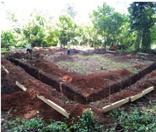
Ongoing construction of toilet facility (ABG)
