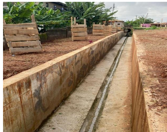
Construction of Storm water drain at Suame
