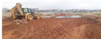
Figure 5: Soil Stabilization Works
