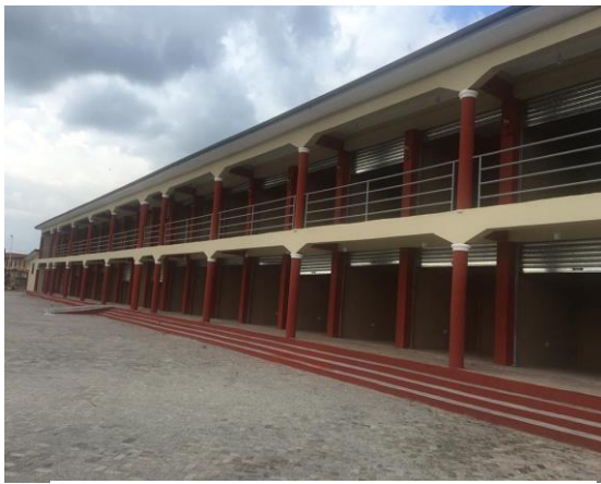
Construction of Market at Berekum East
