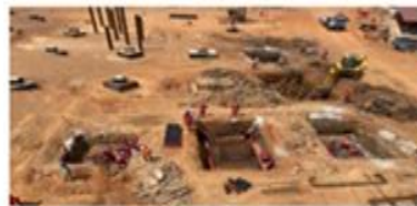
Figure 6: Execution of Pile Caps
