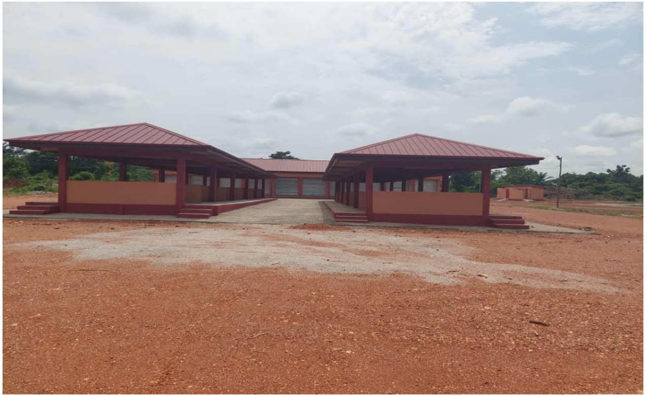
Market shed and lockable stores
