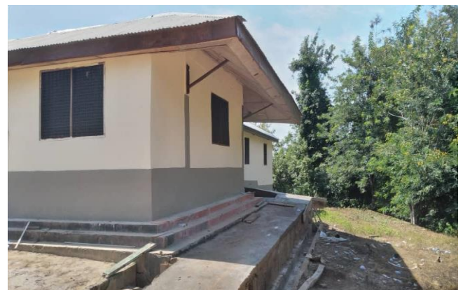
Renovation of Oti Regional Command Office".
