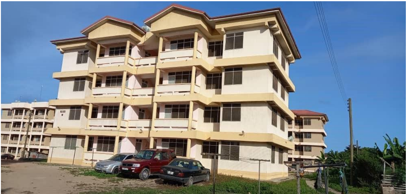
STAFF ACCOMMODATION COMPLETED AT ANKAFU
