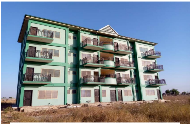
Border Patrol Residential Accommodation at Bawku, Upper East Region
