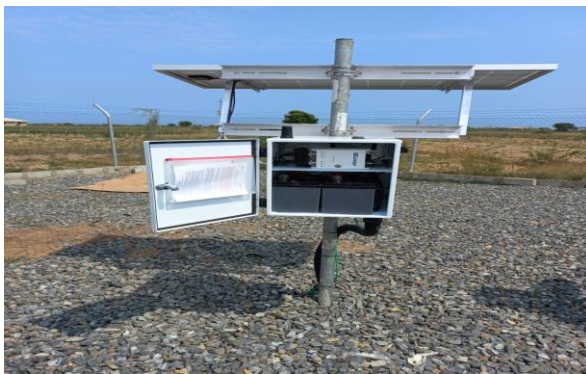
Installation of Seismic equipment
