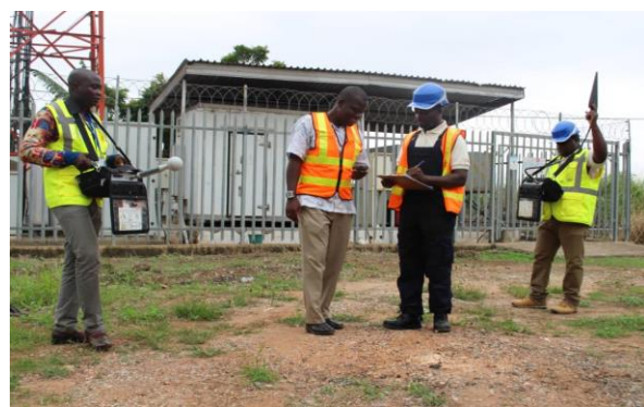
Monitoring of Base Stations
