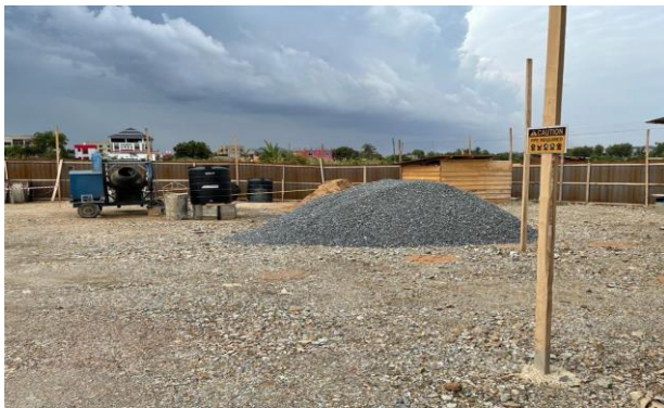
HOC Construction Site
