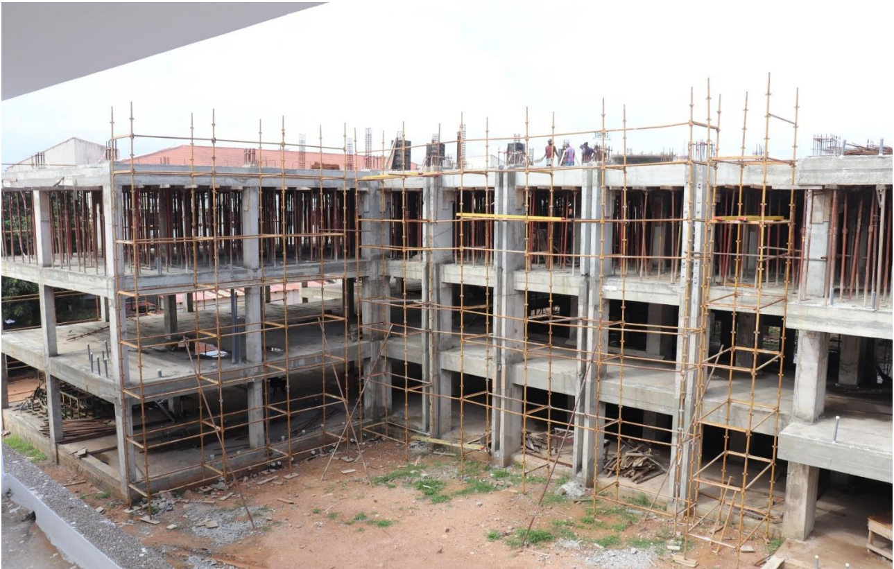
Reconstruction of burnt section of the Old Parliament House – WIP
