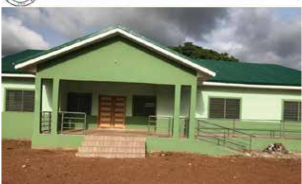
Completed Community Clinic at Zuarungu Community
