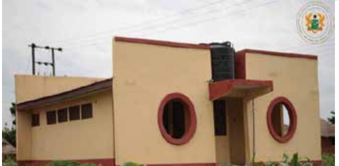
INSTITUTIONAL TOILET AT ZANGBANLUNG KUMBUNGU CONSTITUENCY NORTHERN REGION
