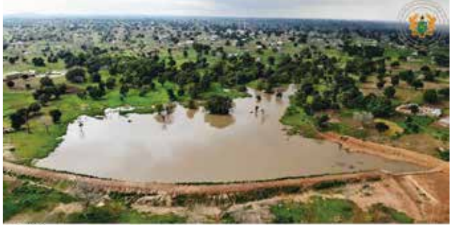
SMALL EARTH DAM, MANYORO, NAVRONGO, UPPER EAST
