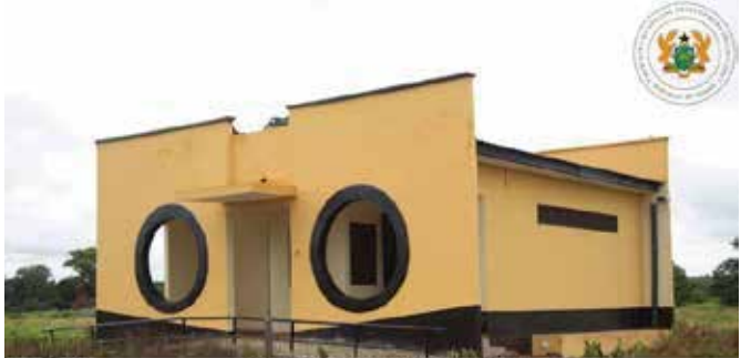
BUNJAI INSTITUTIONAL TOILET SALAGA NORTH CONSTITUENCY SAVANNAH REGION
