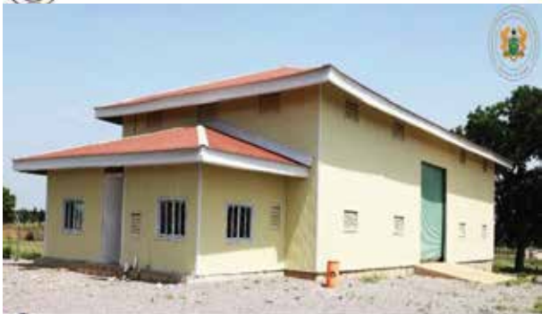
WAREHOUSE, KUMBUNGU, NORTHERN REGION
