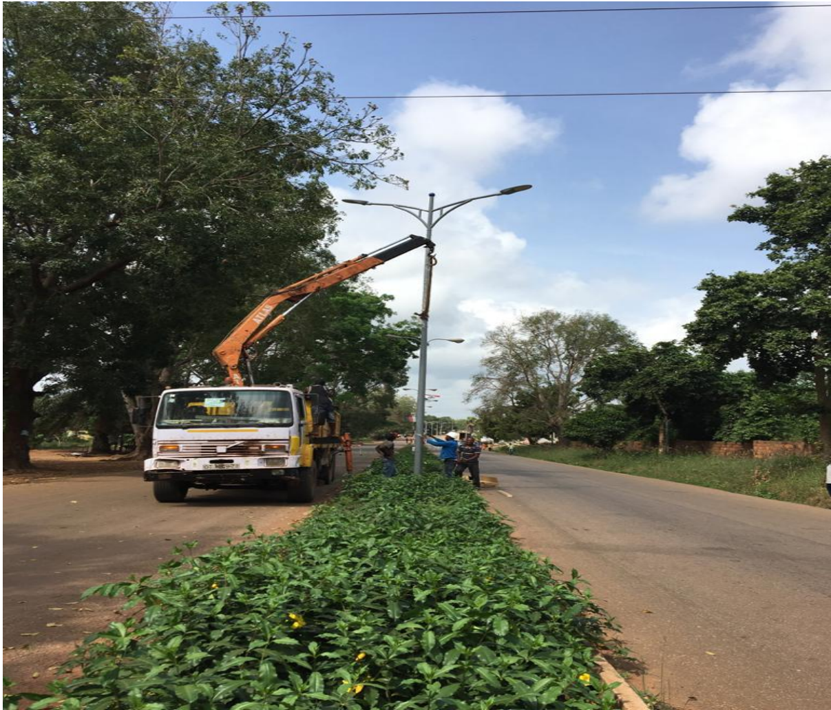
Installation of Street lights
