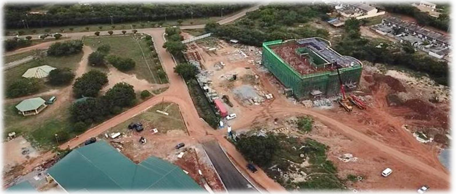
Ongoing Administration Block for Ghana Military Academy
