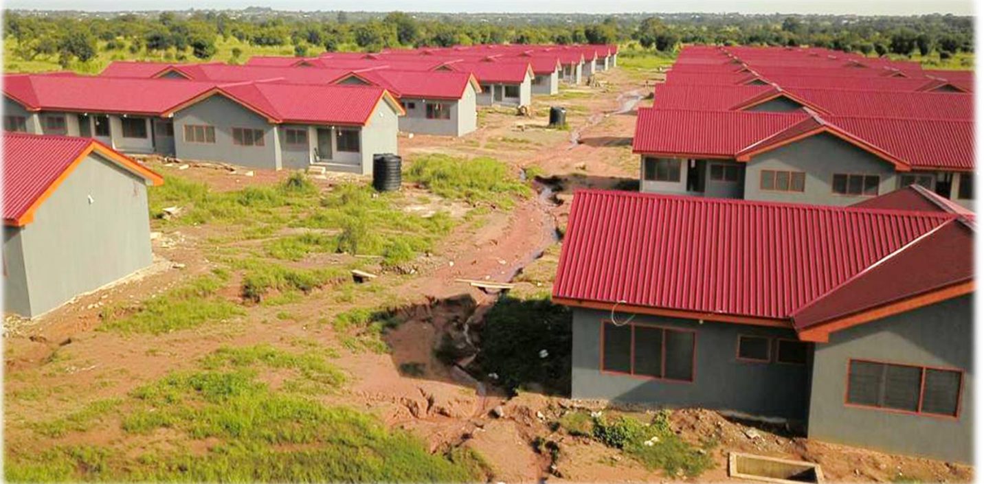
Military Housing Project
