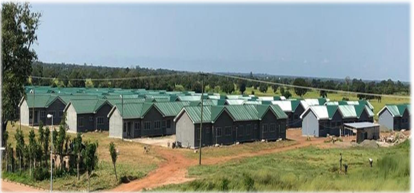
Military Housing Project
