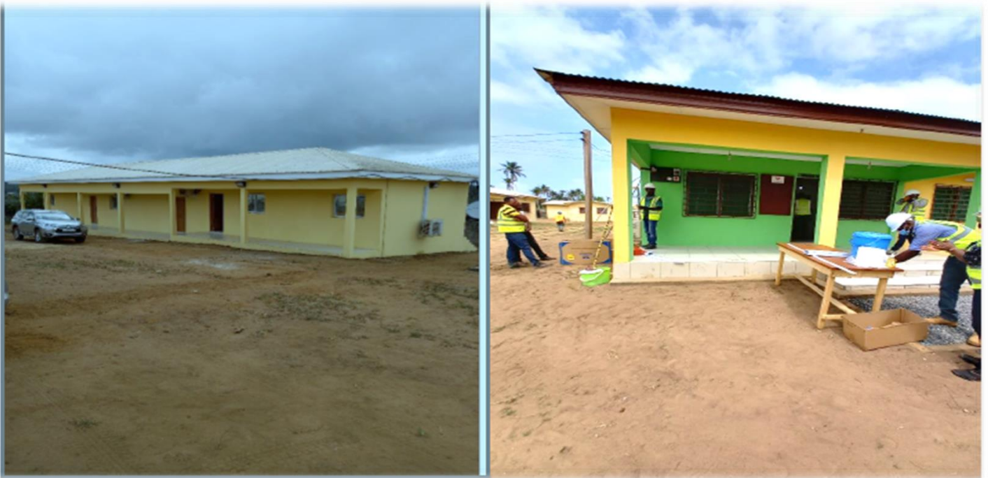
Section of Amandi and Vuluxx Site Office under construction
