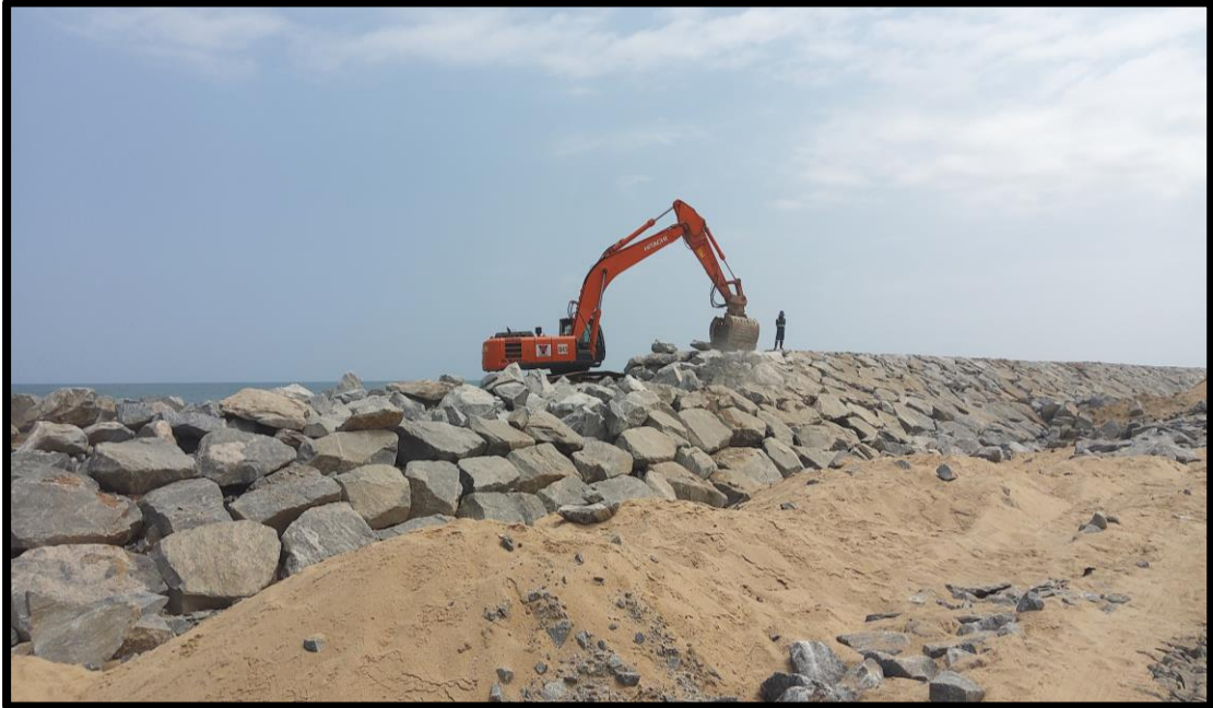
Figure 12: Cape Coast Coastal Protection Project
