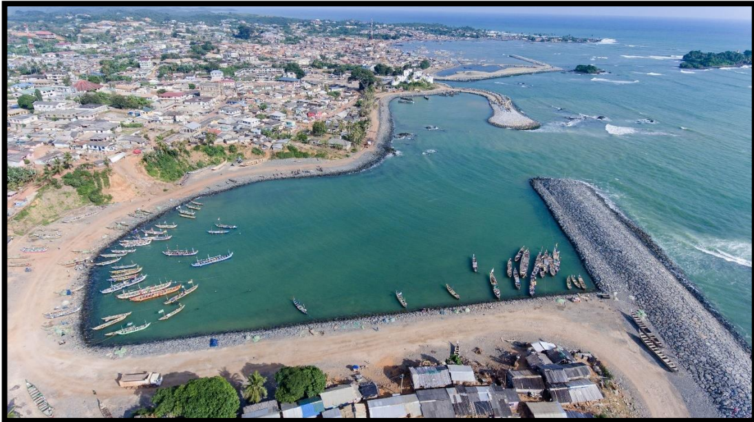
Figure 10: Axim Sea Defence Project
