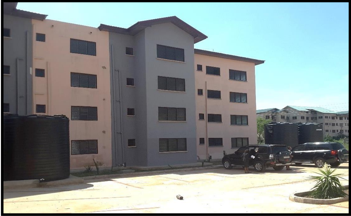
Figure 2: Kpone Affordable Housing Project
