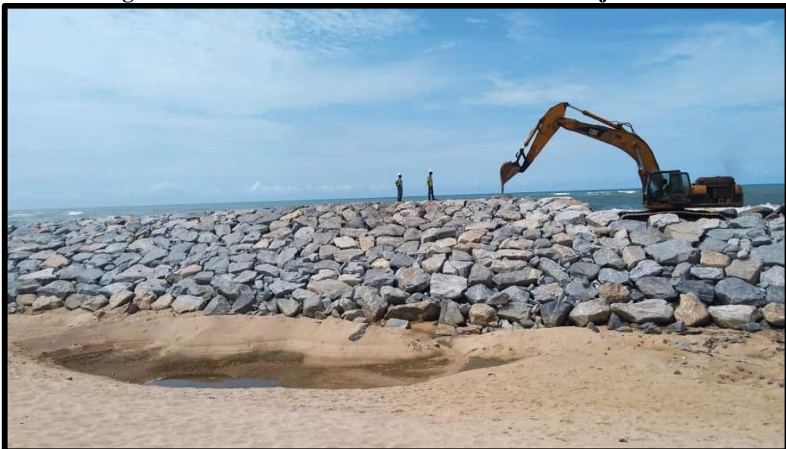
Figure 11: Amanful Kumah Coastal Protection Project
