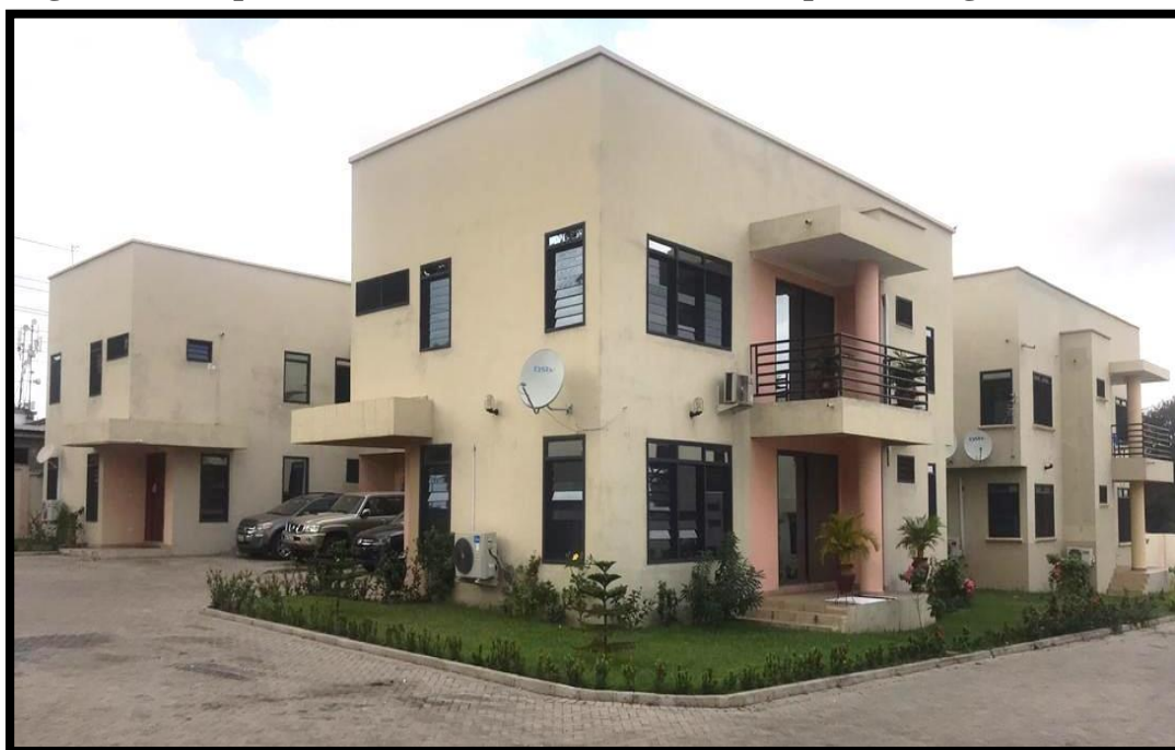
Figure 9: Completed Townhouse under the Redevelopment Programme
