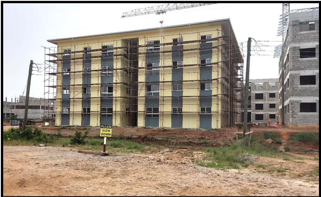
Figure 3: Security Services Housing Project (Phase III)
