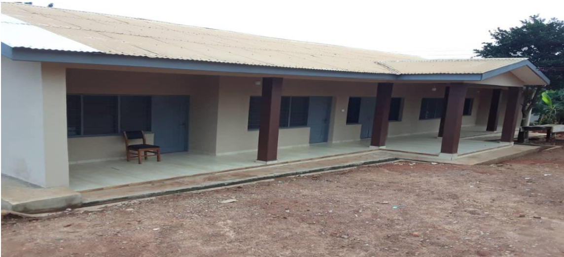
Figure 6 RENOVATION OF GGSA GUEST HOUSE, KUMASI
