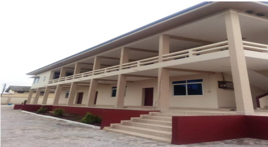
Figure 3 FRONT VIEW OF THE GGSA RENOVATED KUMASI OFFICE BLOCK
