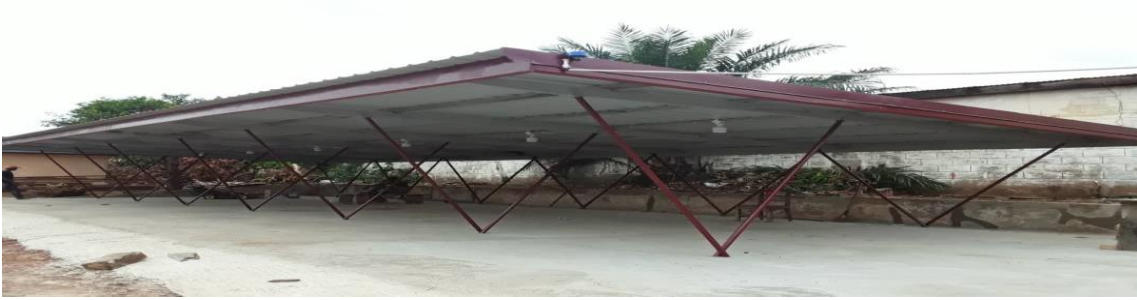
Figure 4 RENOVATION OF GGSA KUMASI OFFICE GARAGE
