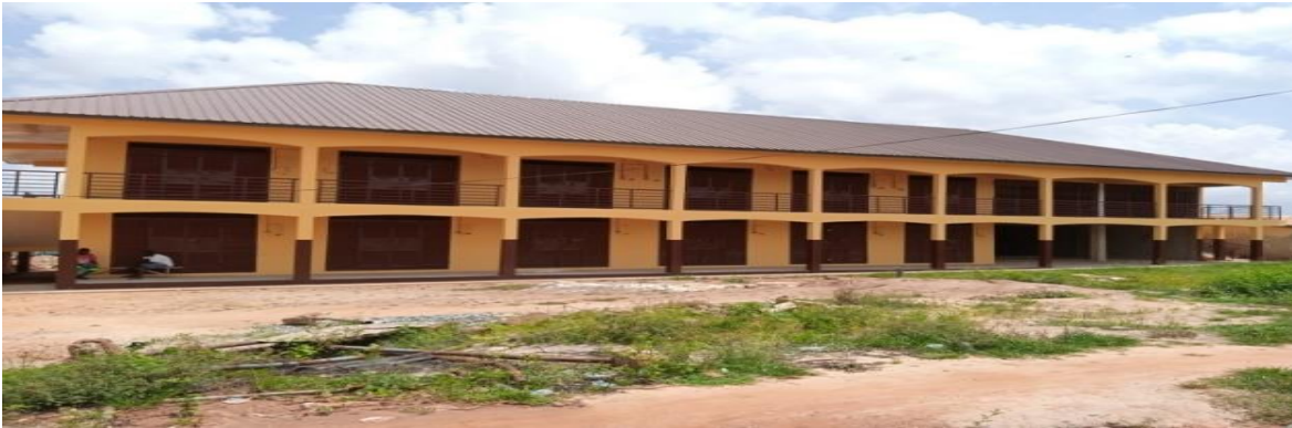
A 32 unit lockable stores at New Abirem
