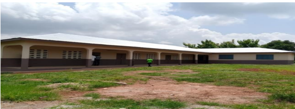
A 3 unit JHS classroom block at Nkwarteng
