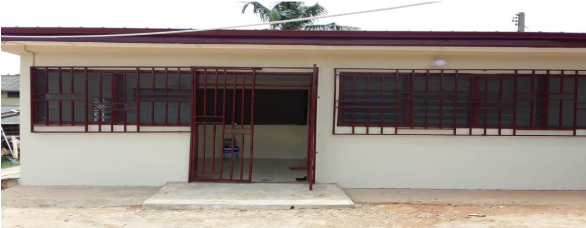
Figure 5 RENOVATION OF KUMASI OFFICE STORE BLOCK
