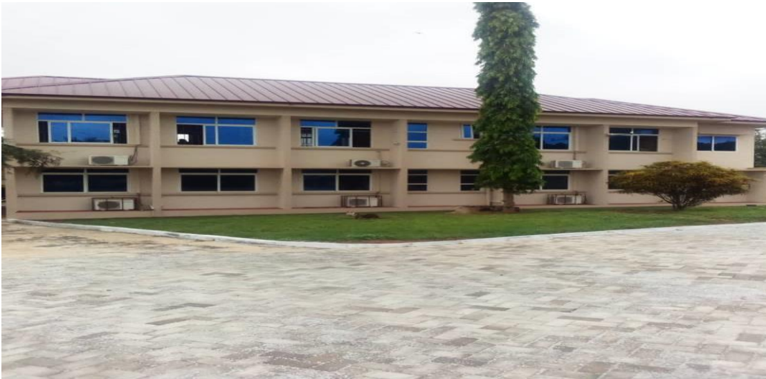
Figure 2 RENOVATION OF GGSA KUMASI OFFICE AND PAVED COMPOUND
