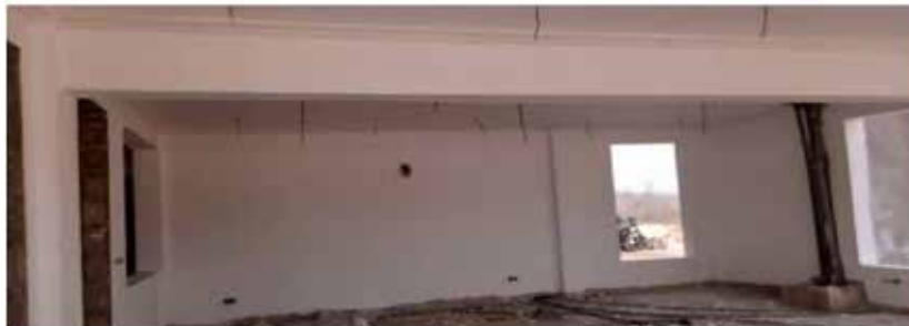
INTERNAL FINISHES ONGOING
