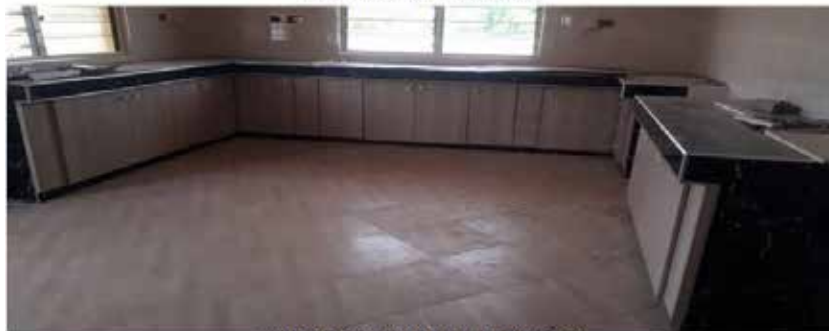
FIXING OF KITCHEN FIXTURES
