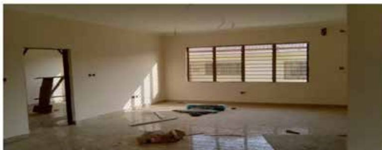
SPRAYING OF FRAMES ONGOING
