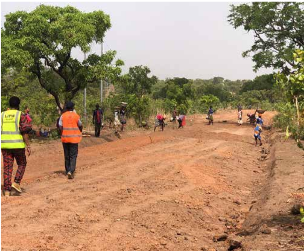
Road works at Derkyi under GSNP
