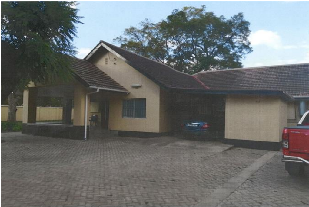
Residence of the Head of Chancery, Ghana High Commission Lusaka, Zambia (Renovated)
