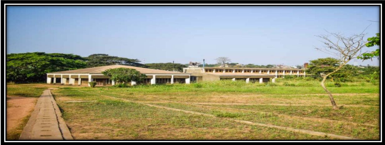
Rehabilitated Auditorium/Canteen Block
