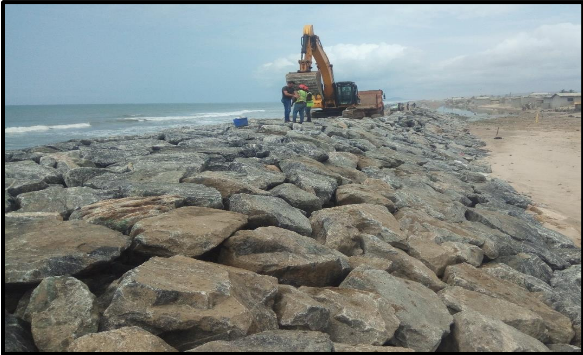
Figure 8: Dansoman Coastal Protection Project
