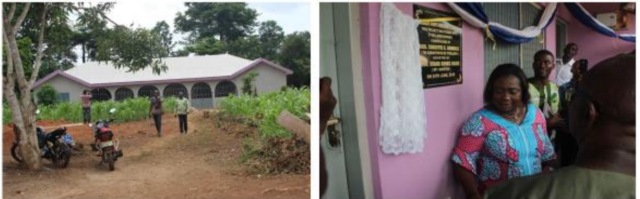
Pomaakrom CHPS Compound with Nurses Quarters – Asunafo North
