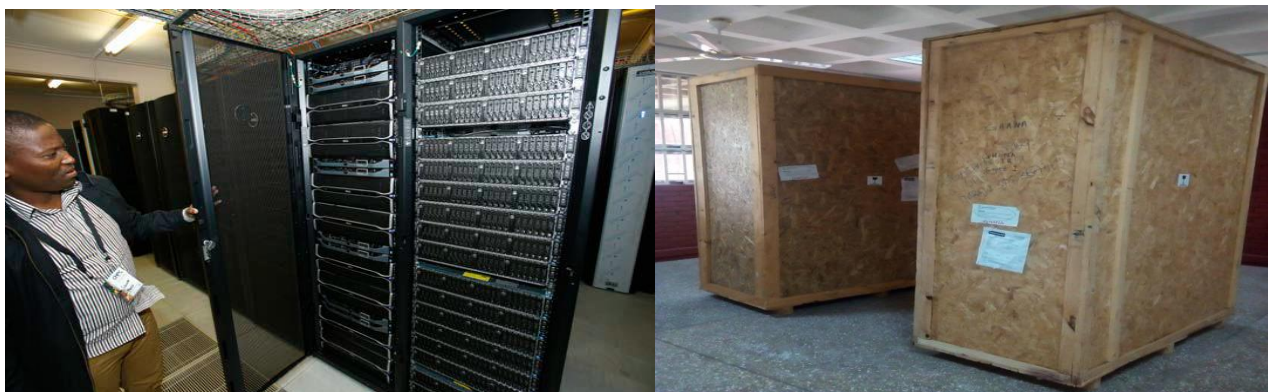
The two Racks of HPC received for the Centre
