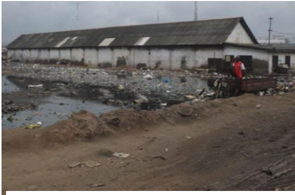
Site before Reconstruction
