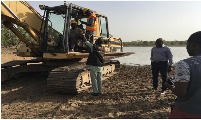
Hon. Minister breaking ground for construction of dam, Kakiase
