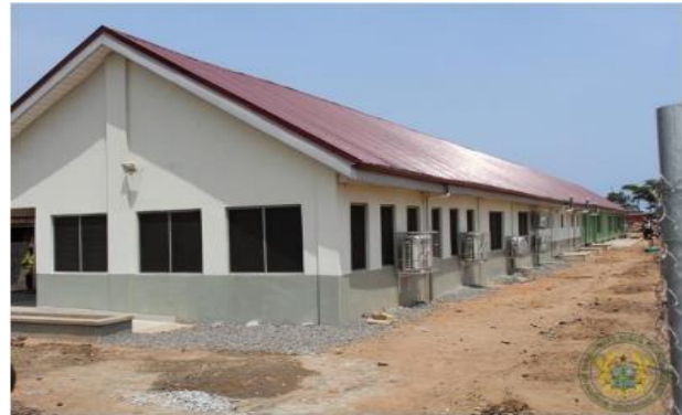
Site after Reconstruction (New Training Facility & Health Post)
