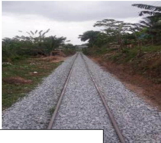
Manual Tamping By GRCL Workers
