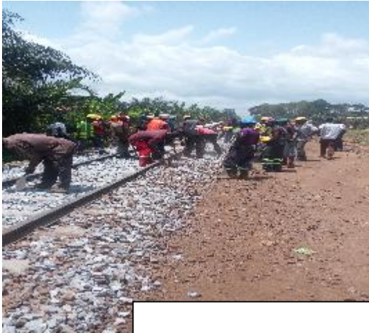
Complete Ballast Track Ready For Tamping
