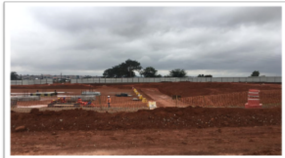
On-going construction of Terminal Building
