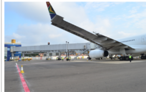
One of No. 6 Installed Aerobridge
