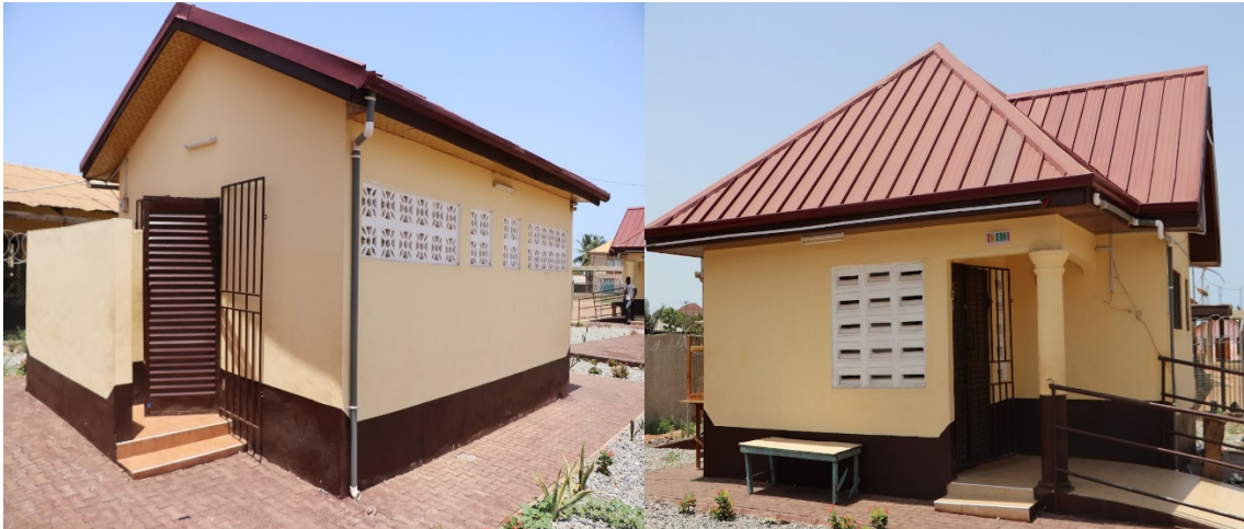
Institutional Latrines under the GAMA water and Sanitation Project
