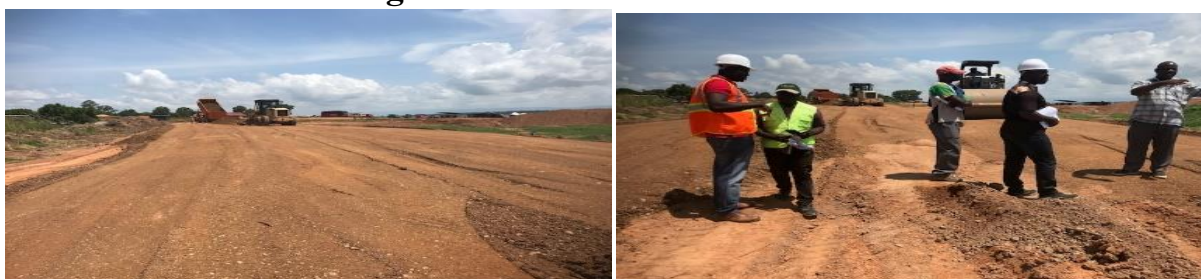
Figure 2: Ongoing Works at Dambai
