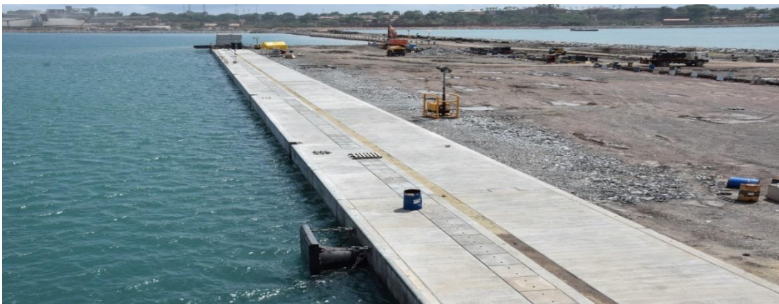
Figure -4: Takoradi Dry Bulk Jetty
