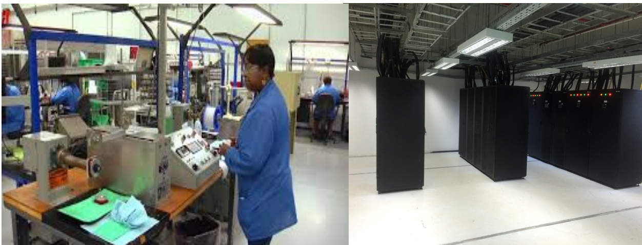
National Data Centre Infrastructure
