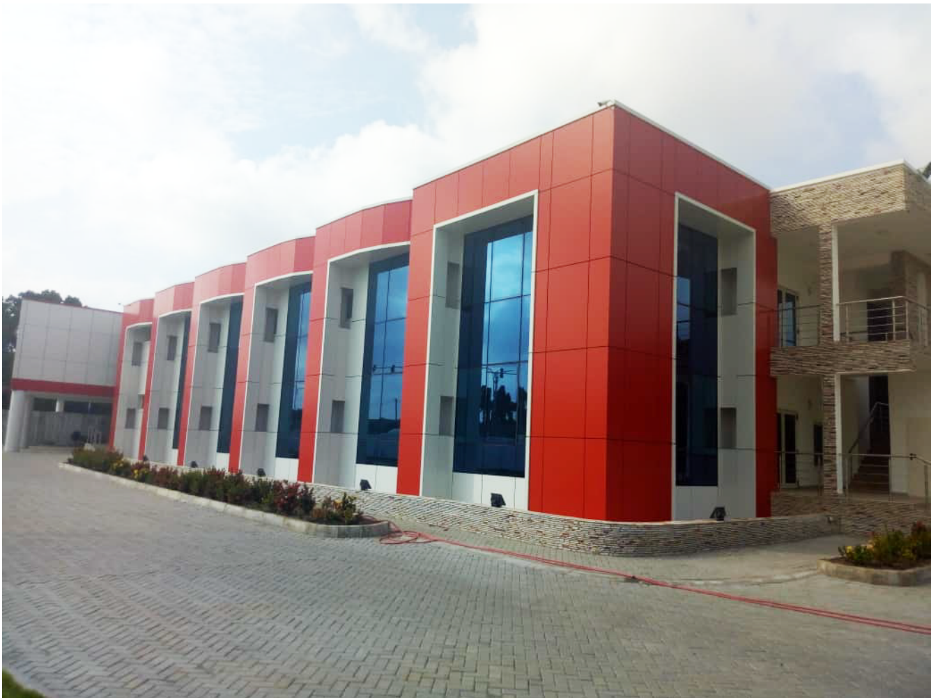
GREATER ACCRA REGIONAL LANDS COMMISSION OFFICE (PHASE 1) IGF FUNDED
