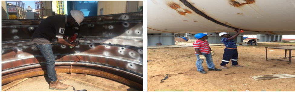
Welding using NDT Techniques
