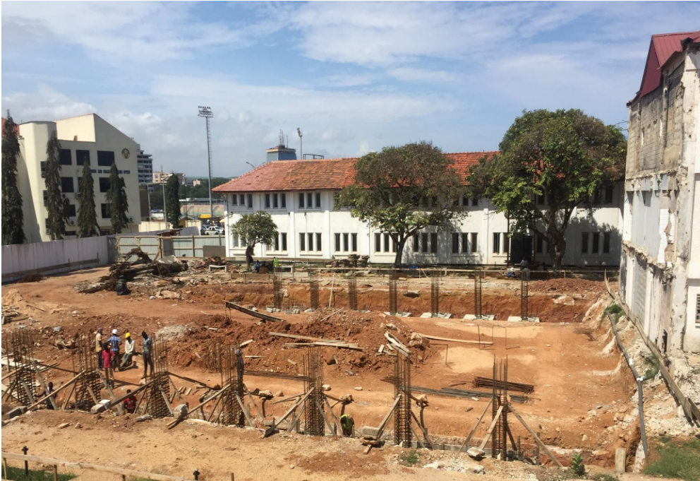
Reconstruction Work commences at the Old Parliament House, High Street
