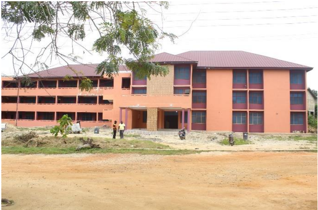
CONSTRUCTION OF 2 – STOREY 1 NO. NEW ASSEMBLY BLOCK AT SHAMA
