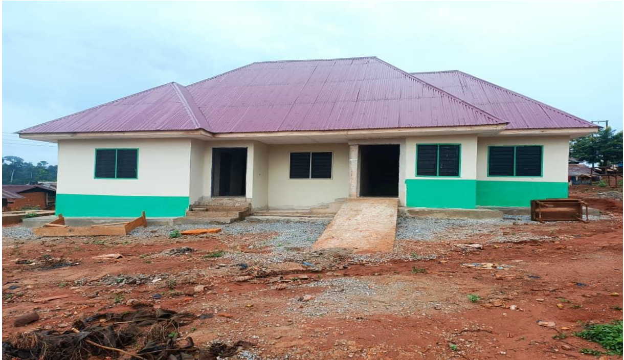
Construction of 1No. CHPS at Juaboso Nkwanta
