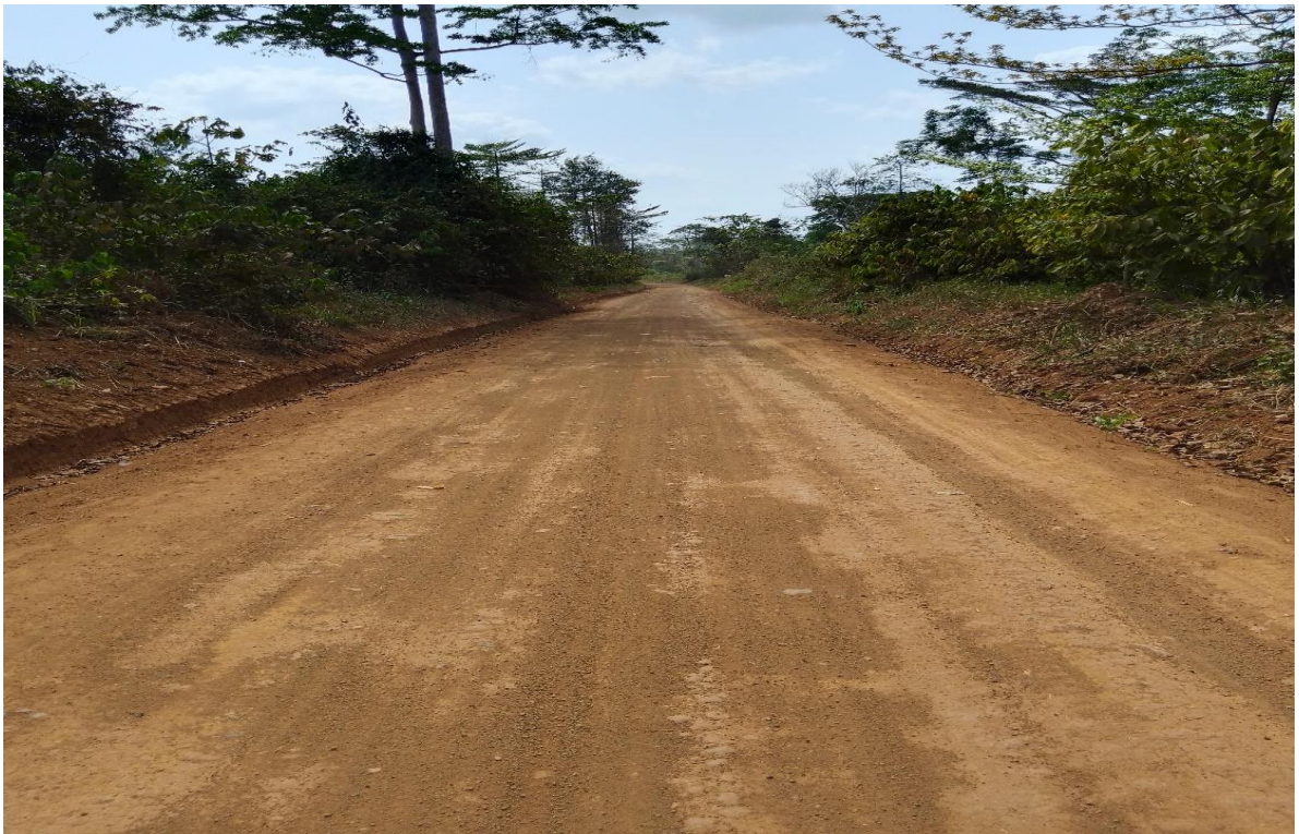
Reshaping of Krokosue to Asempaneye Feeder Road
