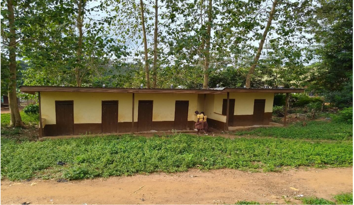
Construction of 1No. 6 Seater VIP Toilet at Juaboso Cluster of Schools
