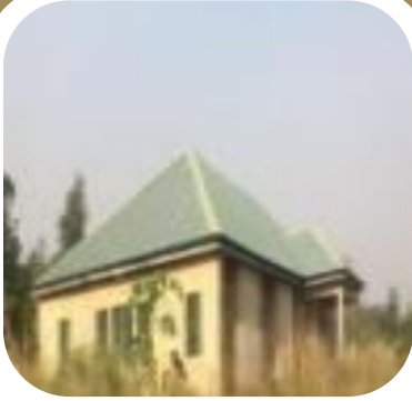
Completion of Medical Consultants Bungalow at Akatsi.
