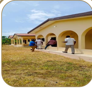
Completed 1 No 4-Unit Nurses Quarters at Wute, and it has been handed over for use.
