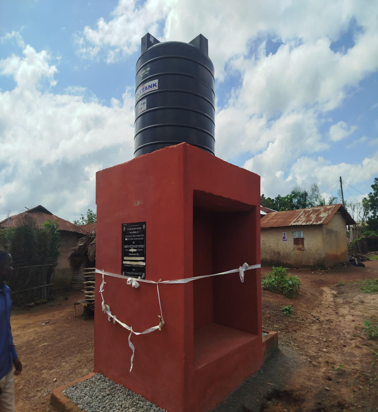
Drilled 1No. Mechanized Borehole with Storage - Poly Tank at Dzadzape
