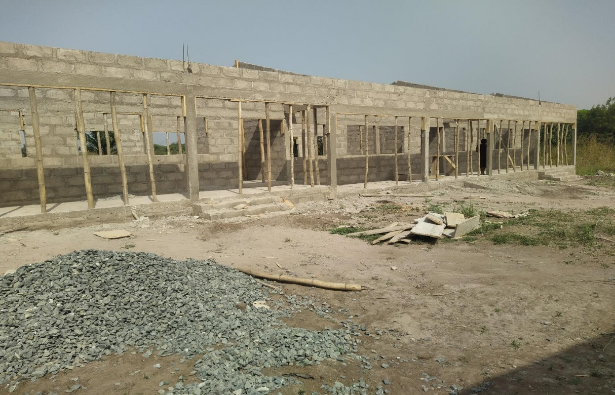
Construction of 1No. Classroom Block with store at Adaklu Vodze - DACF
