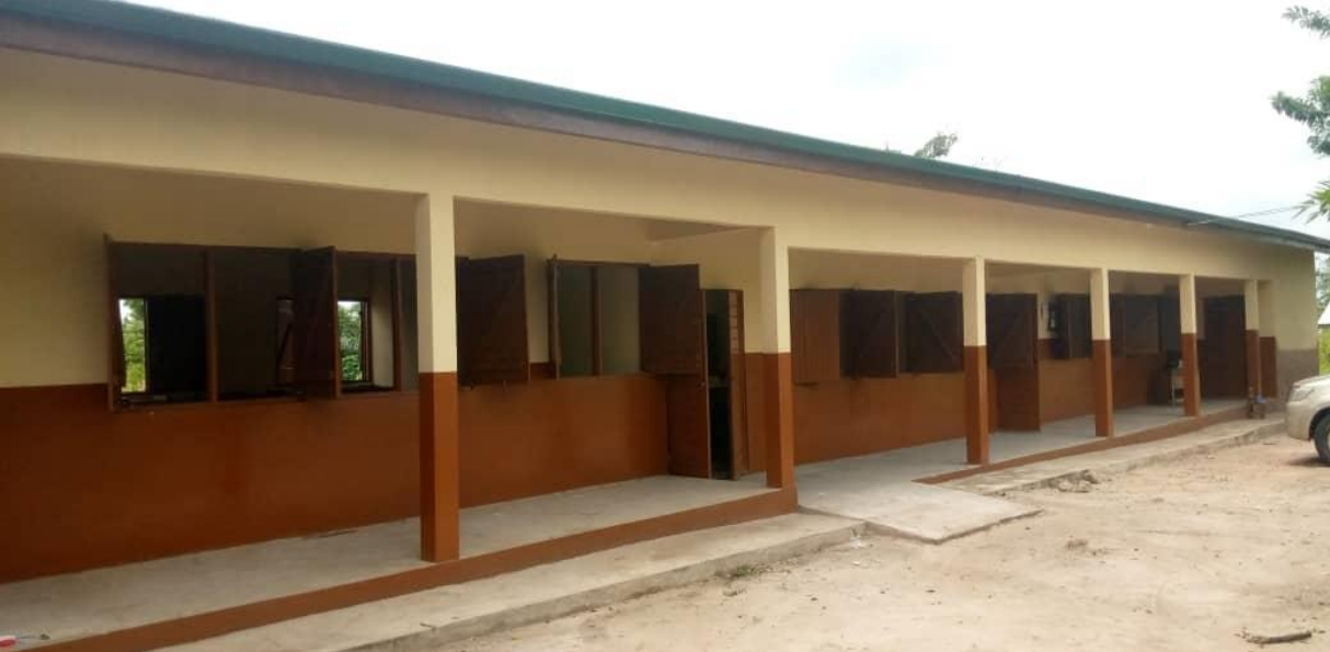
Completed 1No. 3unit Classroom Block at Adaklu Tavikpo (DACF)
