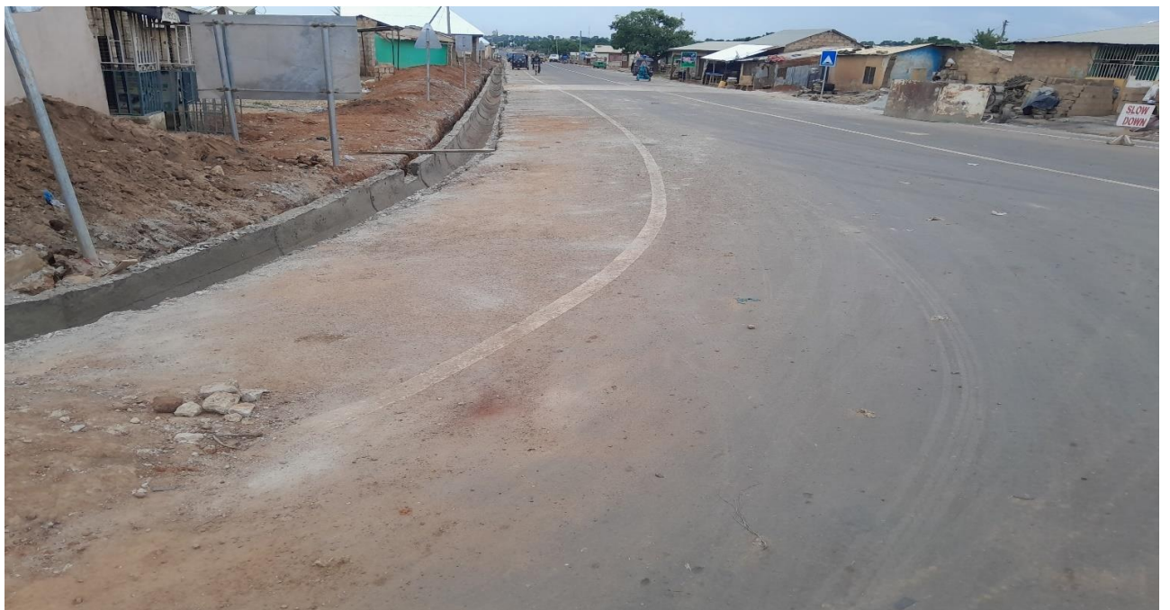
Wa-charia Road Constructed.
