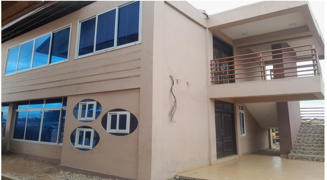
Town Hall And Restaurant Constructed
