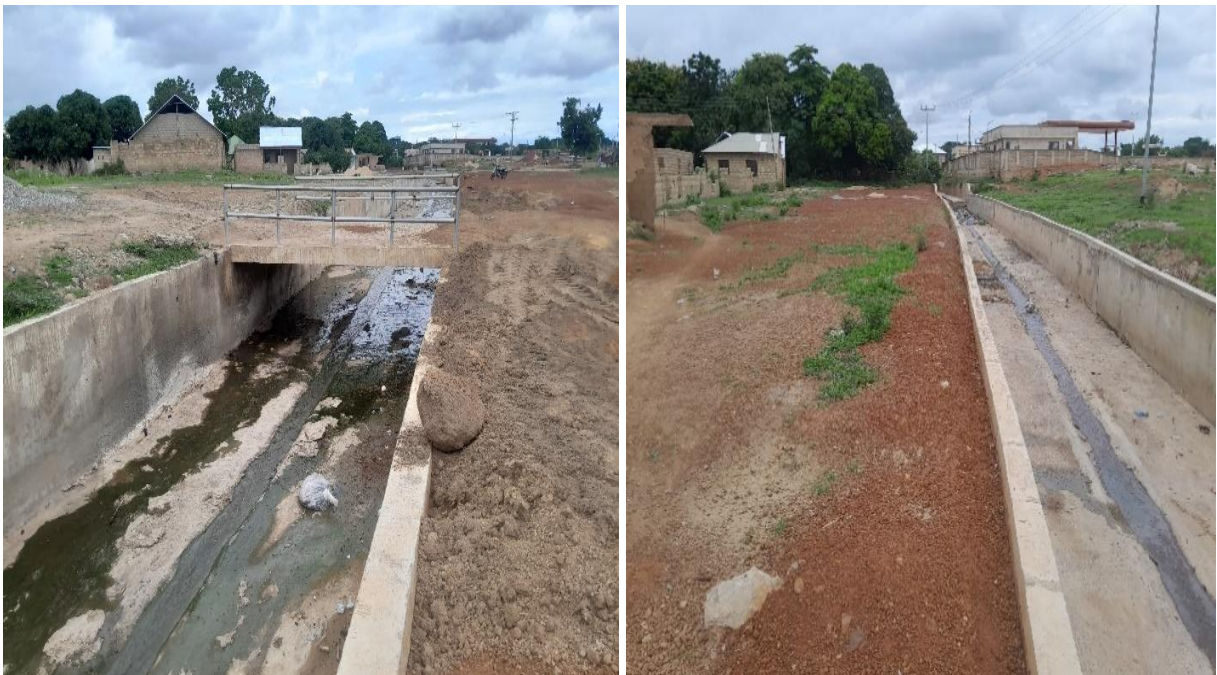
Concrete Storm Drain Constructed at Kambali.
