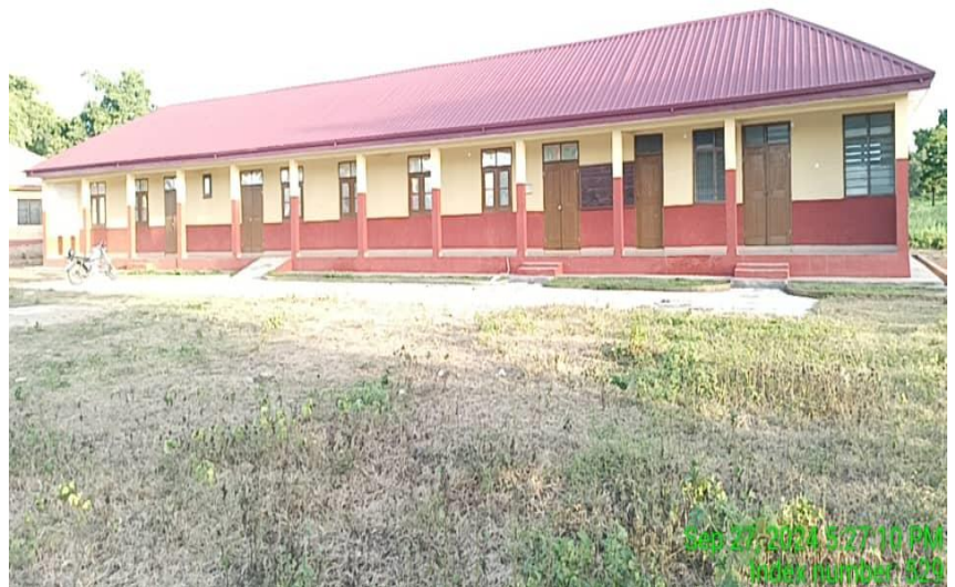
Completed 1No 3-Unit Classroom Block with Furniture at Jawia Muabelle (funding SOCO)
