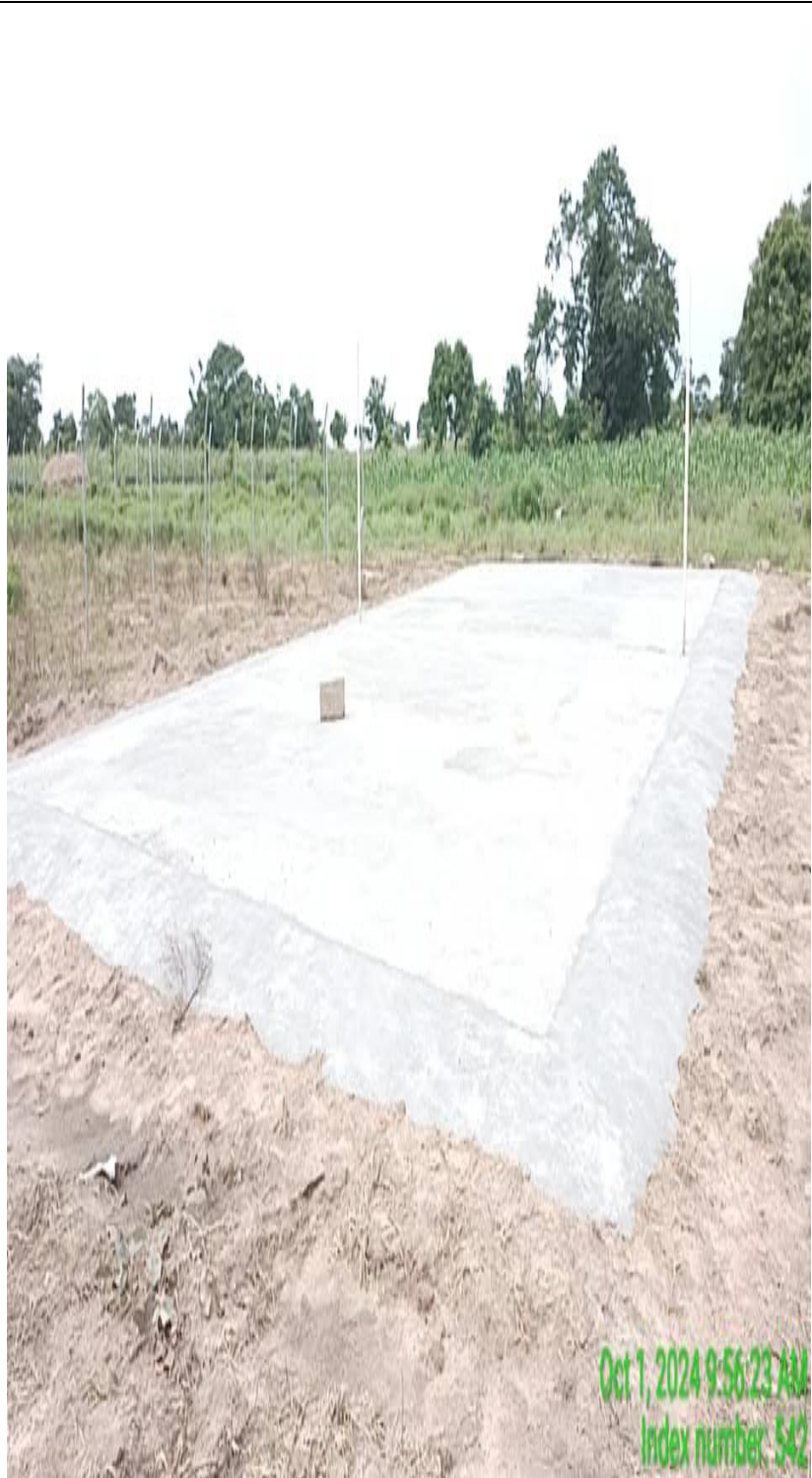
Construction of Football and Volleyball Fields in Gwollu (SOCO)
