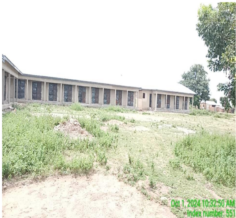
Construction of Market Stalls at New Gwollu Market ( Funding SOCO)
