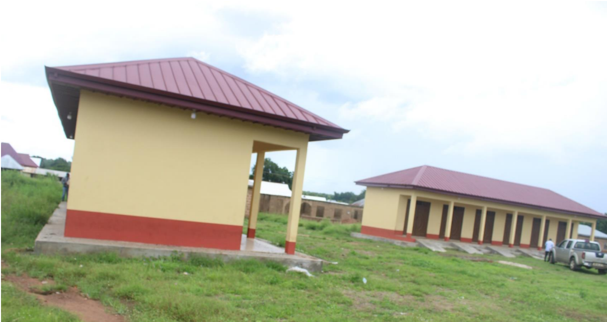
Construction 1no. 6unit Lockerable Market stores at Naro and Nanvilli
