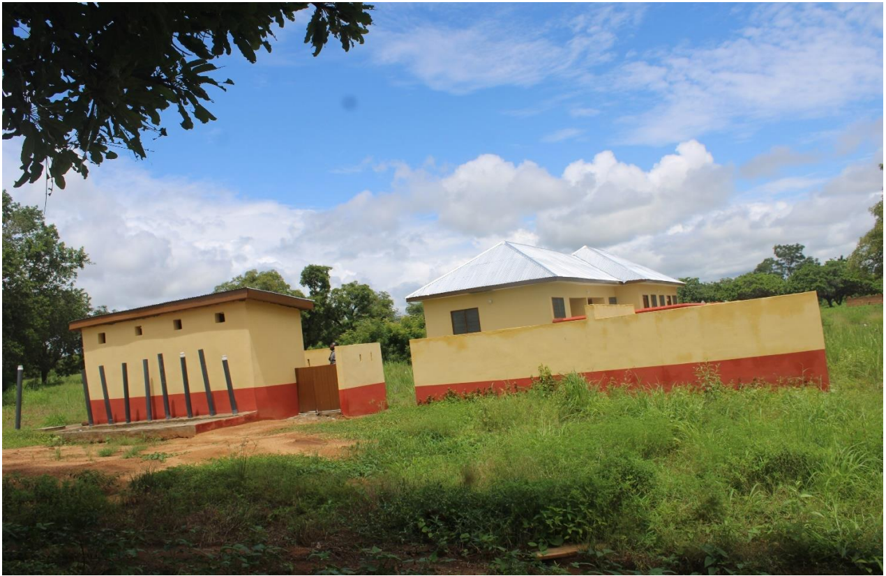
Constructed 1no. CHPS Compound at Nator-Duori
