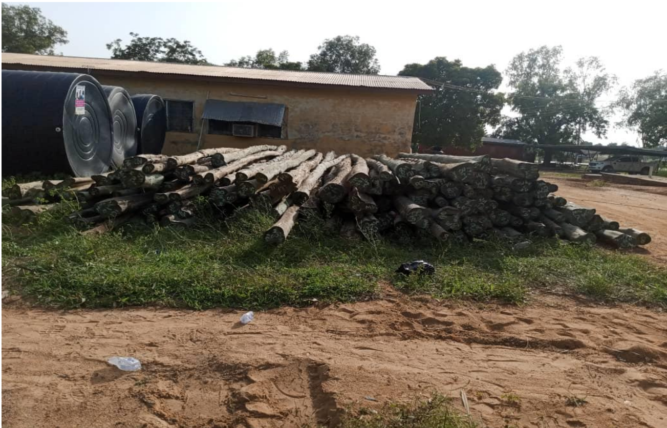
Supplied 192 8-Meter low tension poles District wide
