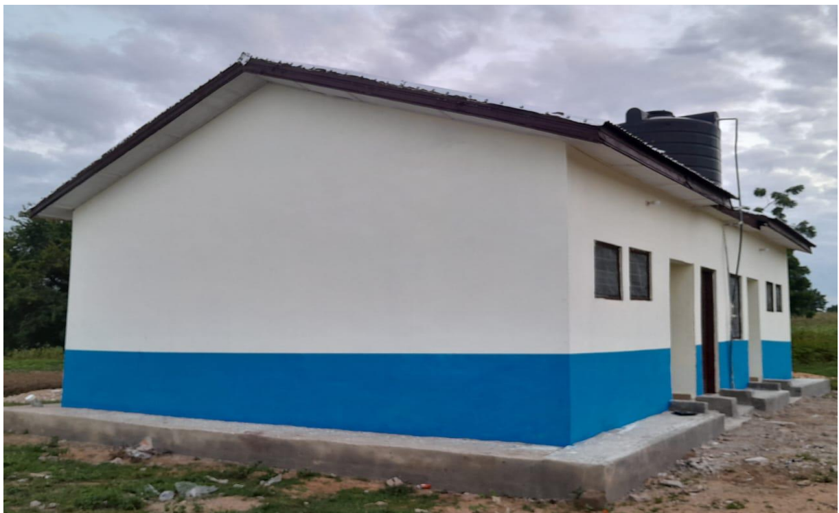
1no. Pour Flush Completed at Tubong
