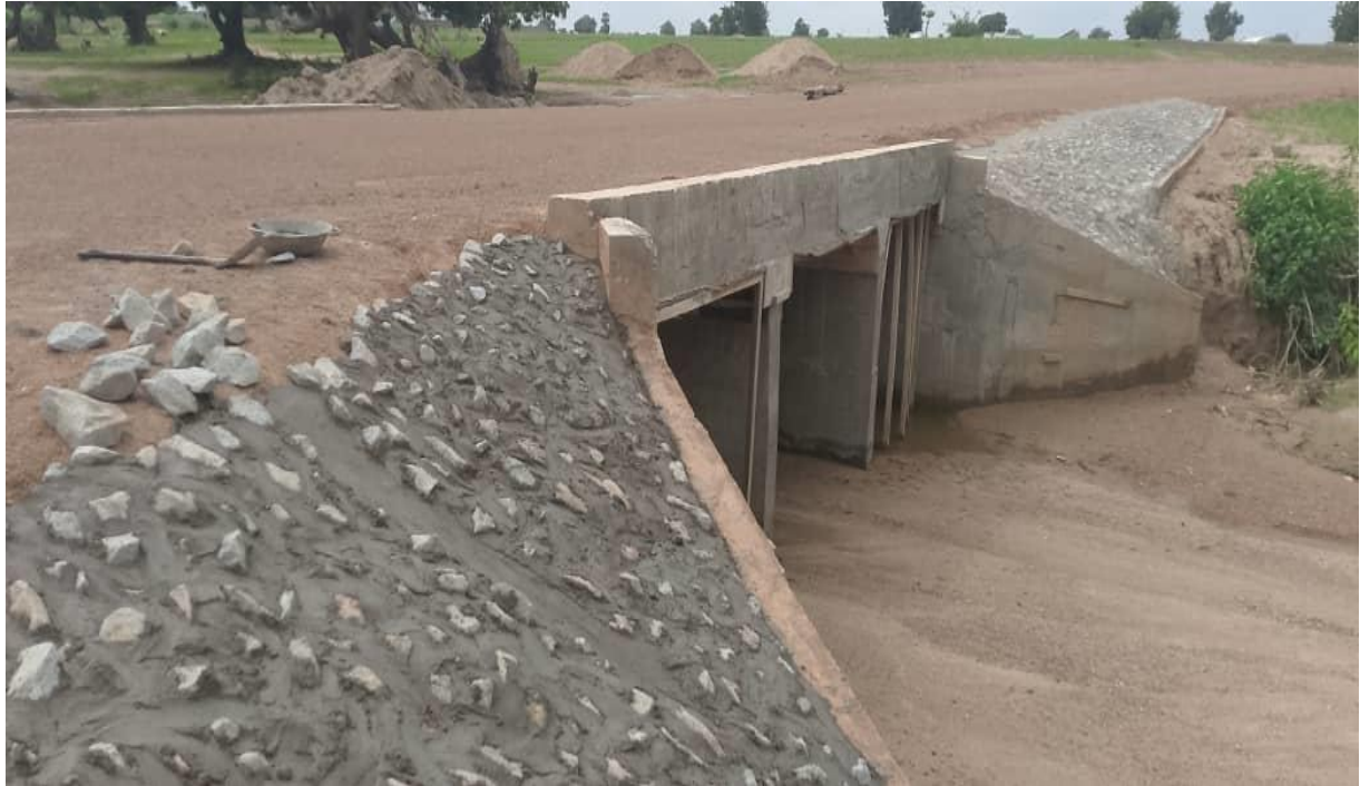
Completed 3mx3m Box Culvert at Tafpkuan
