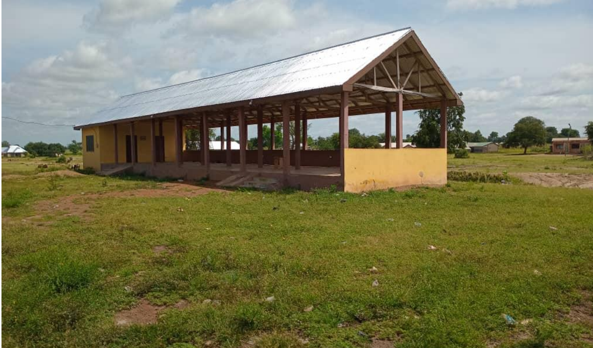
Constructed 1NO 8-Unit Market Sheds and 2NO Market Stalls at Pelungu-SOCO
