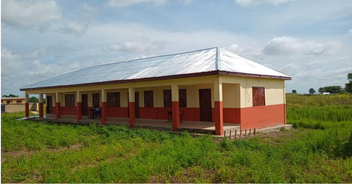
Constructed 3-unit classroom block with head teachers' office and a store at Soliga DACF-MP.
