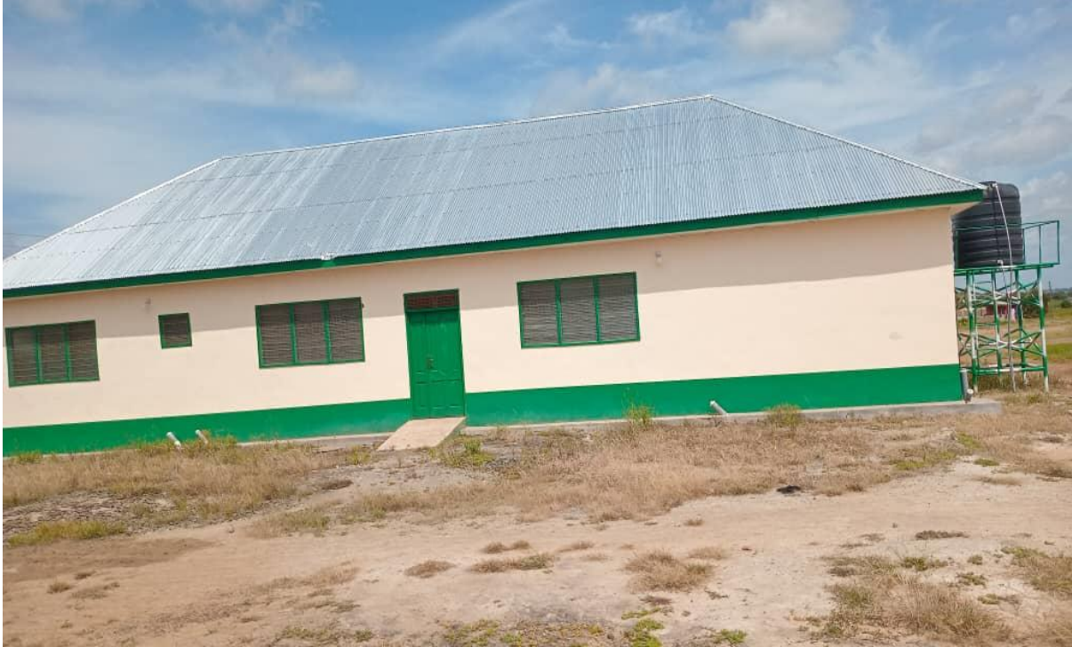
Constructed 1No. 3-Unit maternity block at Pelungu Heath Center-SOCO
