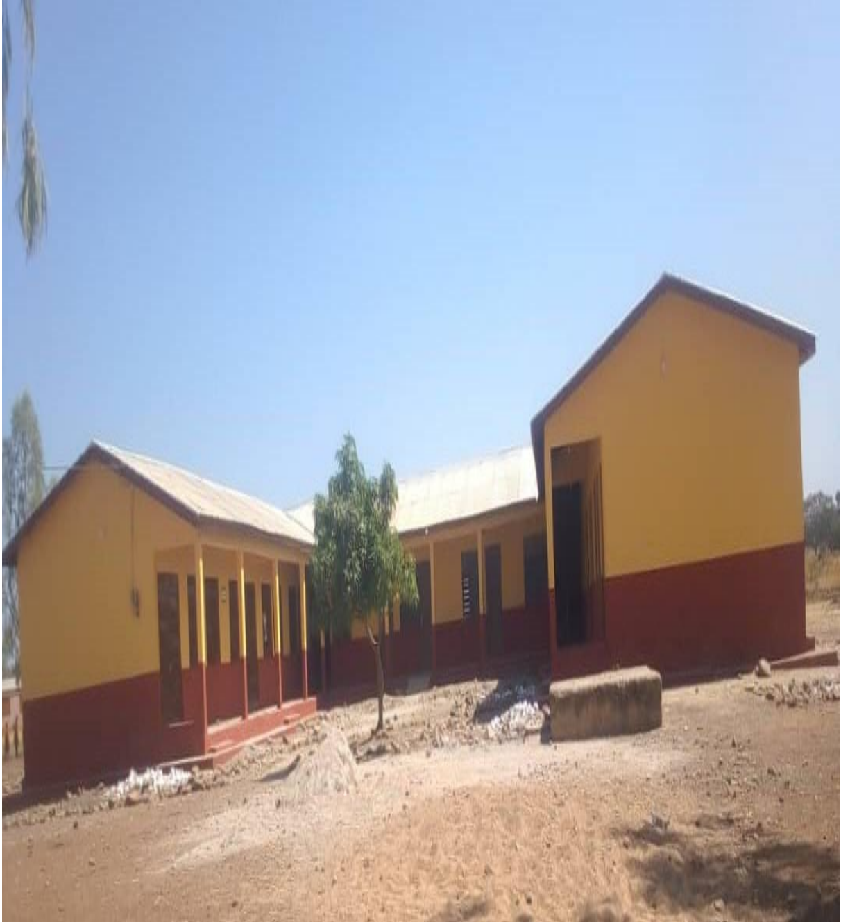
Rehabilitated 6-unit classroom block at Dagliga-SOCO
