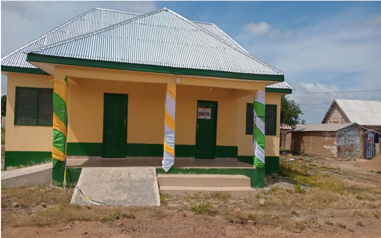
Constructed 1No. 2-Unit maternity block at Pelungu Heath Center-NPA
