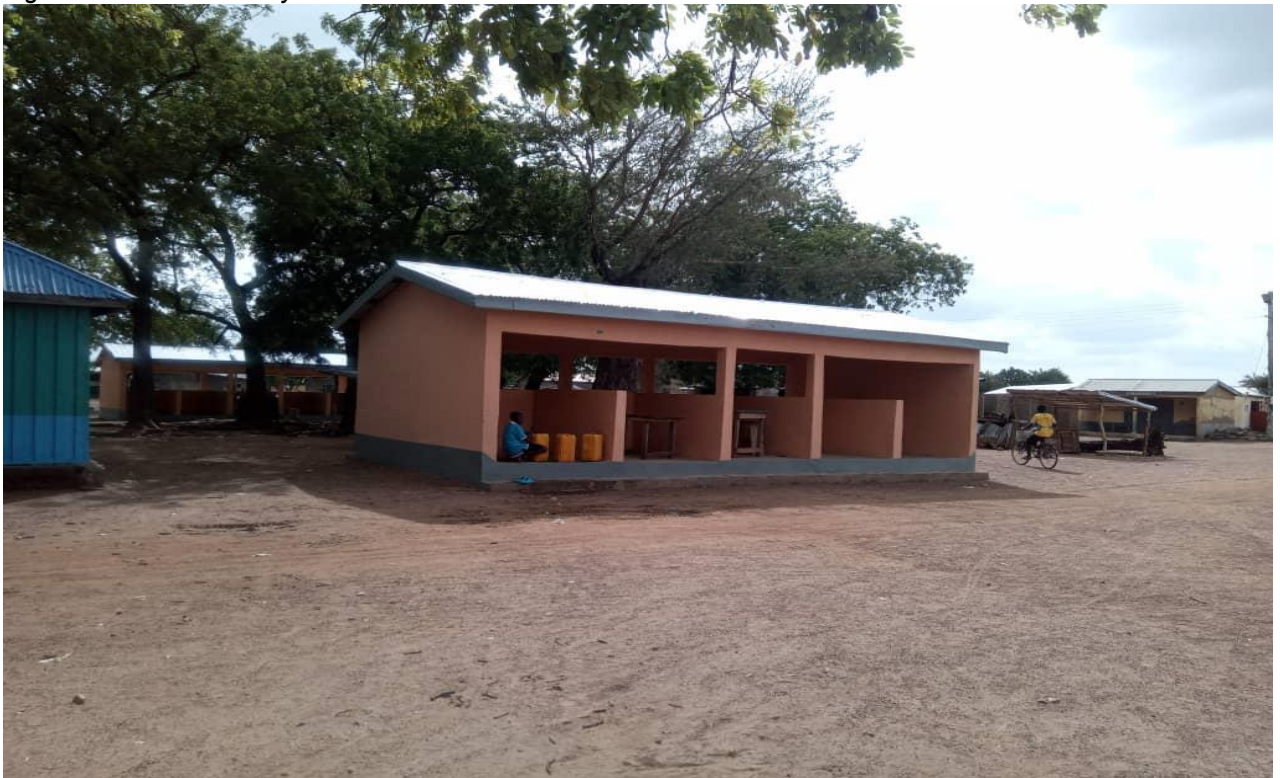
Constructed 10No. Market stalls at Kanjarga
