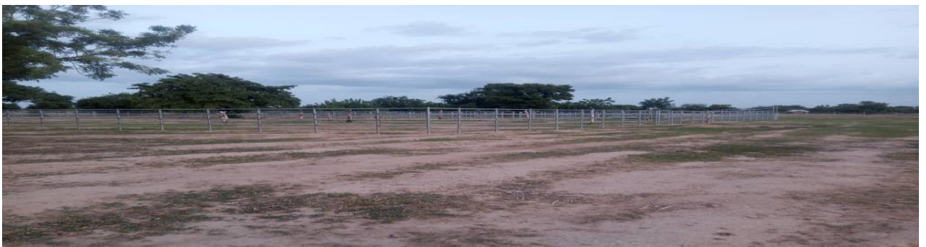
Constructed and Fenced 1No. Animal Market with 3no. offices at Fumbisi
