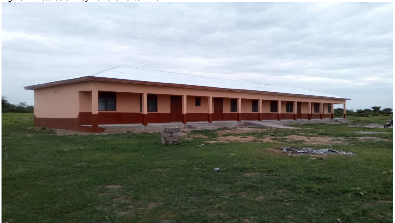
Construction of 1No. 3-Unit Classroom block at Logvosa
