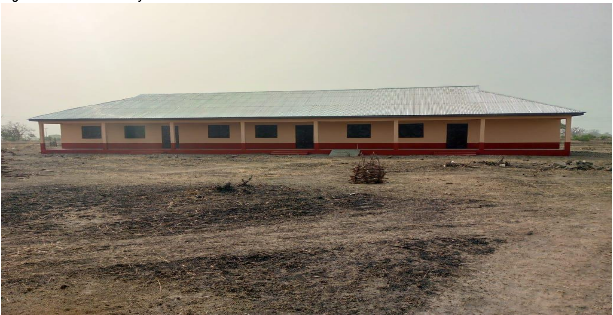
Constructed 1No. 3-Unit classroom block at Kaseisa
