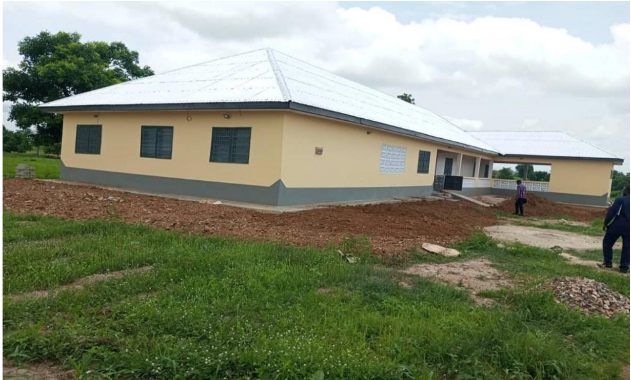
Constructed 1No. CHPs compound with nurses' accommodation at Dabore
