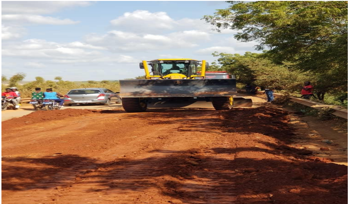
Spot improvement of Kolaa bridge section of the Bolga-Bawku road
