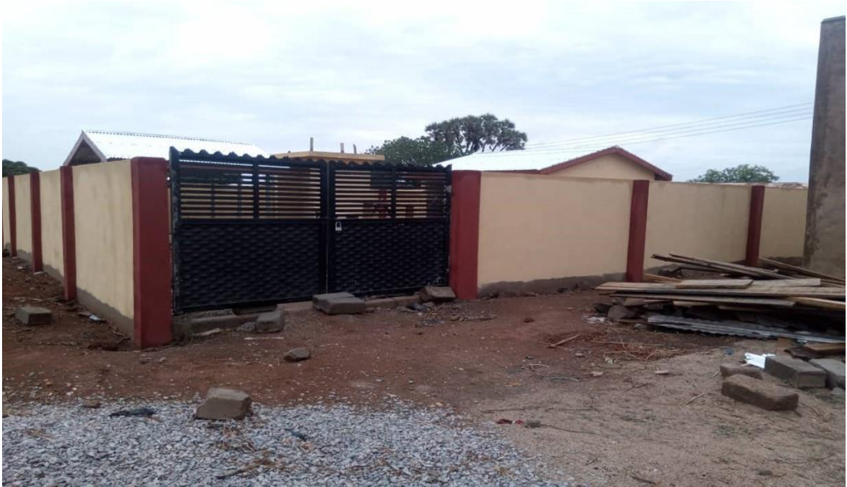
Rehabilitated 1No 10-seater toilet facility with overhead tank at Zuarungu market
