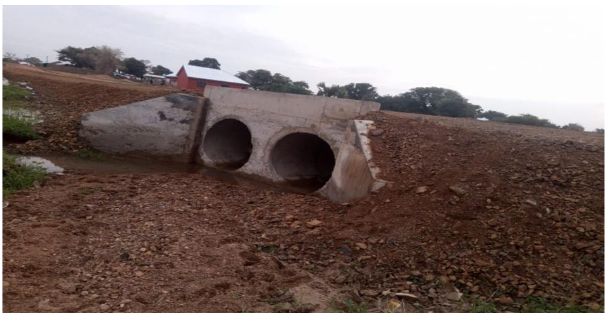
Constructed 1No culvert with 6-metre width at Kumbosigo
