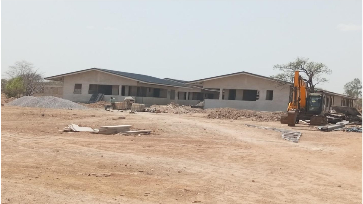
Construction of Agenda 111 hospital project at Katanka
