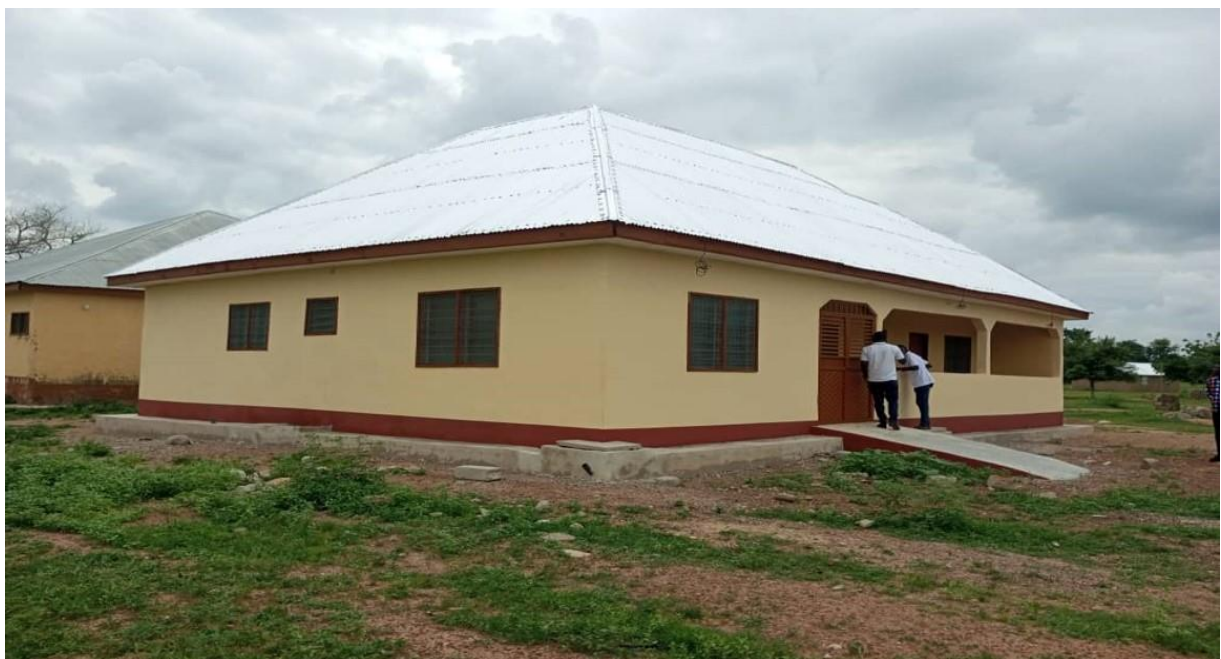
Constructed 3-unit accommodation for nurses at Dulugu CHPS compound
