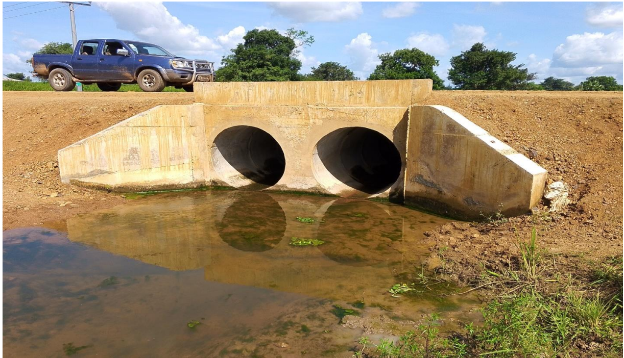
Constructed 1No culvert with 6-metre width at Dachio
