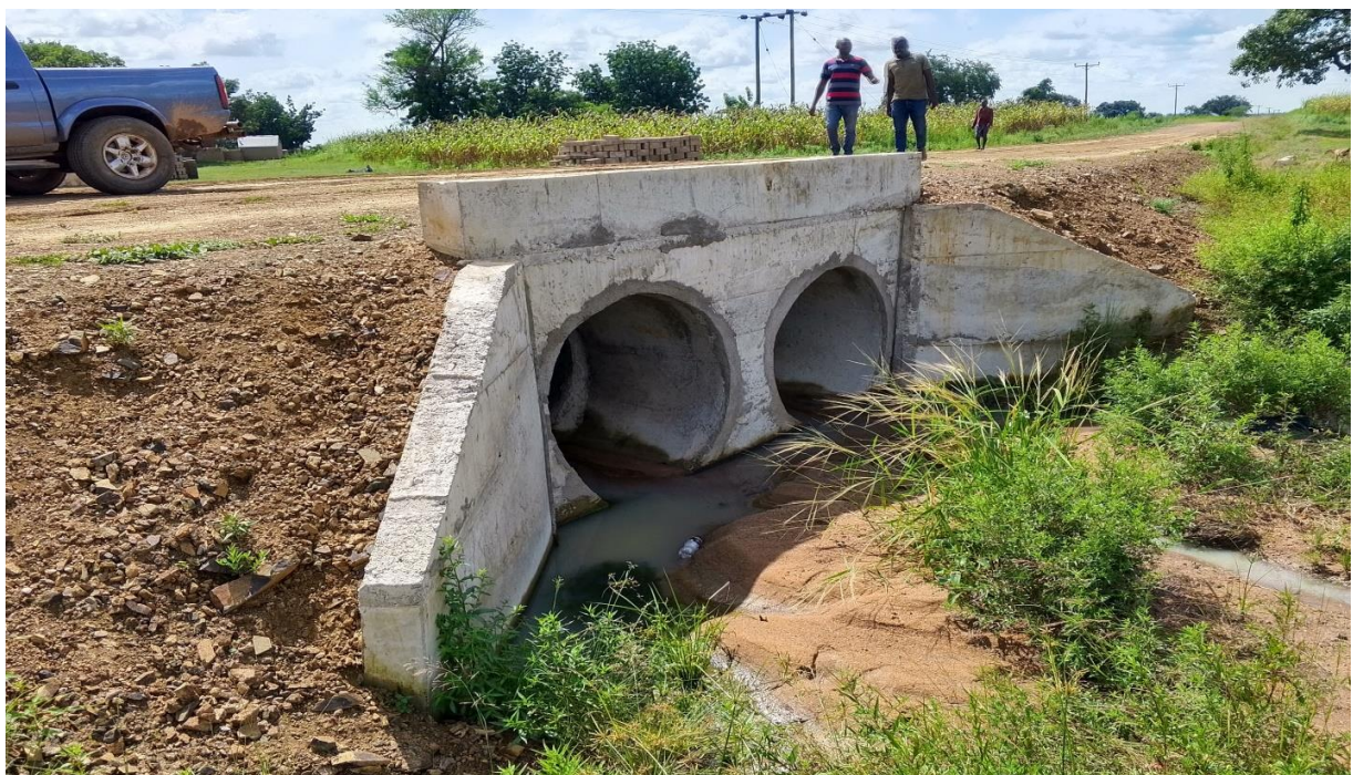
Constructed 1No culvert with 6-metre width at Zonno-Zori
