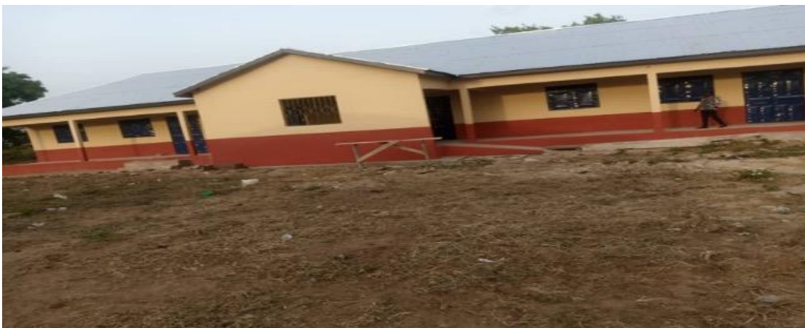
1 no. 3 unit classroom block constructed at Sori 2
