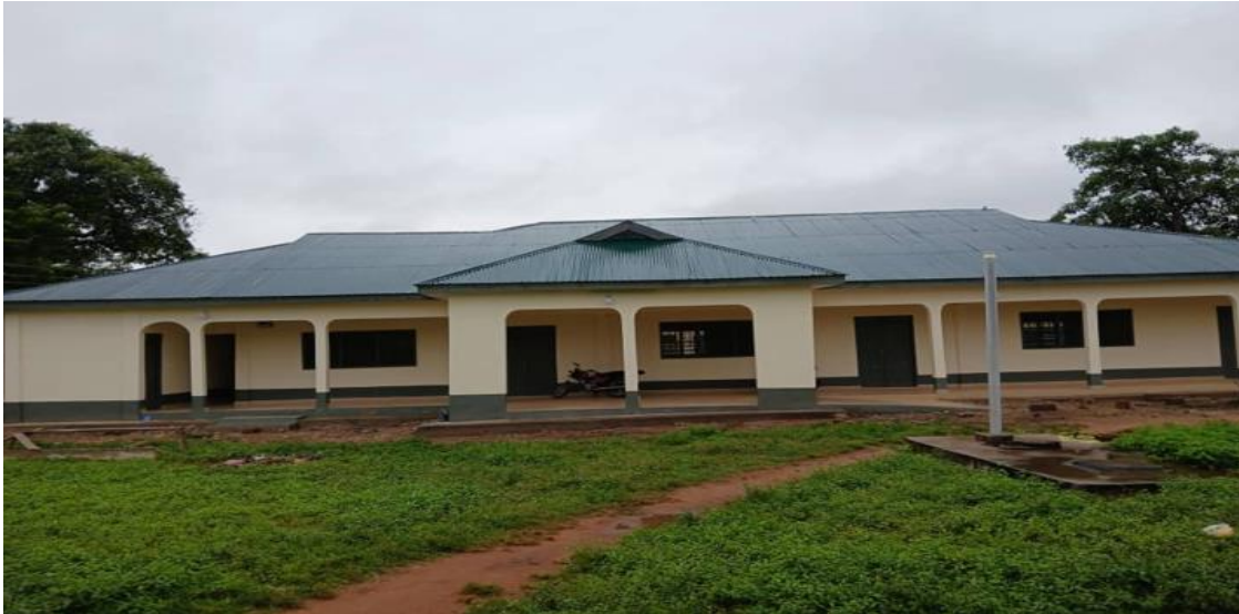
1 no. Lecture Hall constructed at Damongo nursing and midwifery training school.
